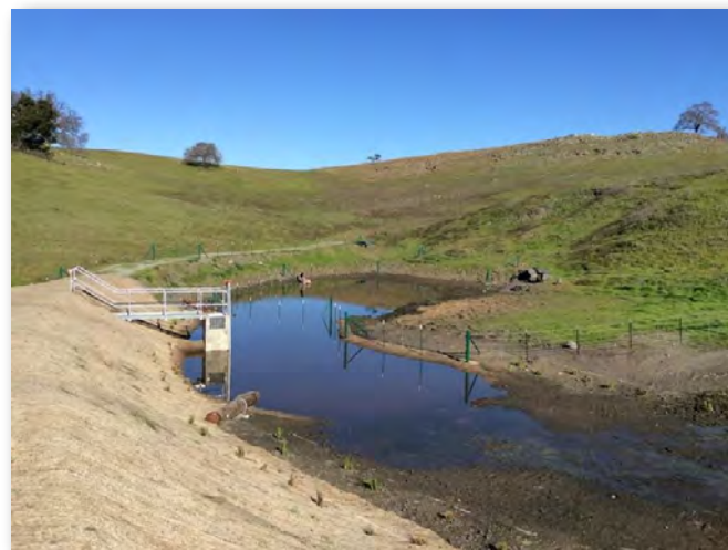
Photo 4. Post construction conditions at the Pond Site (December, 2016)
