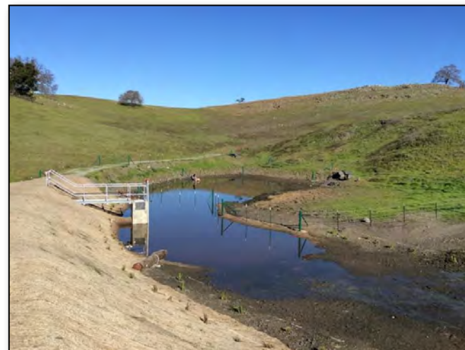
Photo 2. Post construction conditions at the Pond Site (December, 2016)
