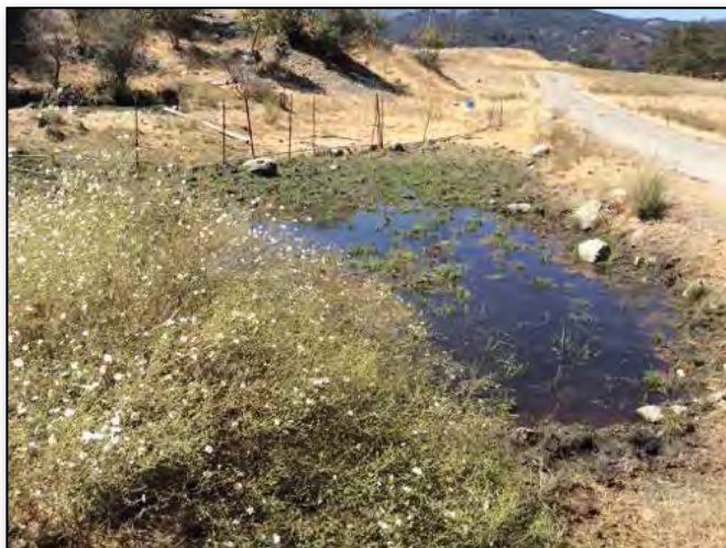
Photo 1. Preconstruction conditions at the Wetland Mitigation Site (August, 2016)
