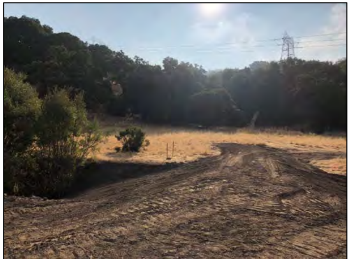
Post-Treatment Irrigation Ditch Channel Plug ED03-04
