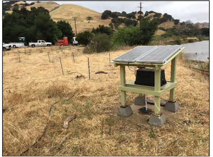
Solar Pump irrigation system
