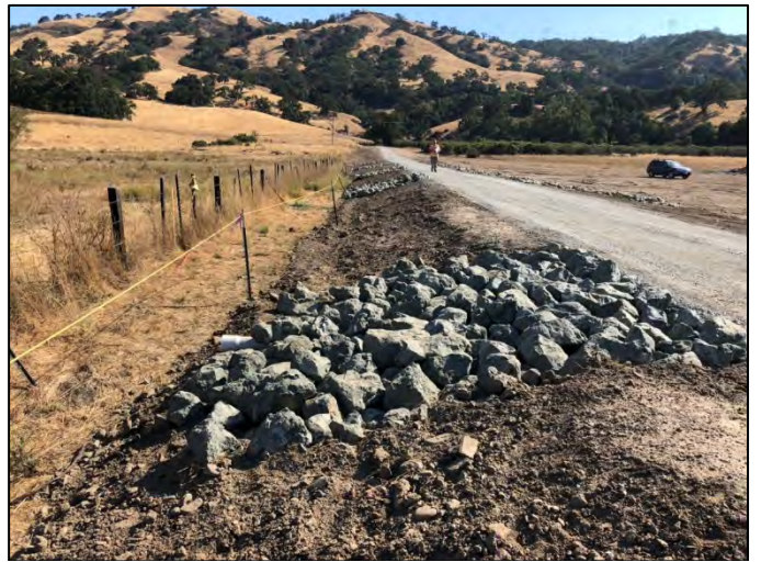
Post-Treatment Corral Trail Drainage Lenses R-01
