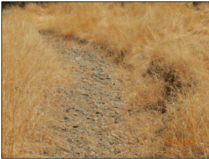
Pre-Treatment Boyd's Creek Main Stem at Fifth Log Structure ID01-01
