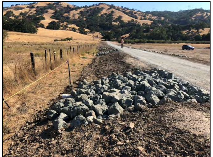
Post-Treatment Corral Trail Drainage Lenses R-01
