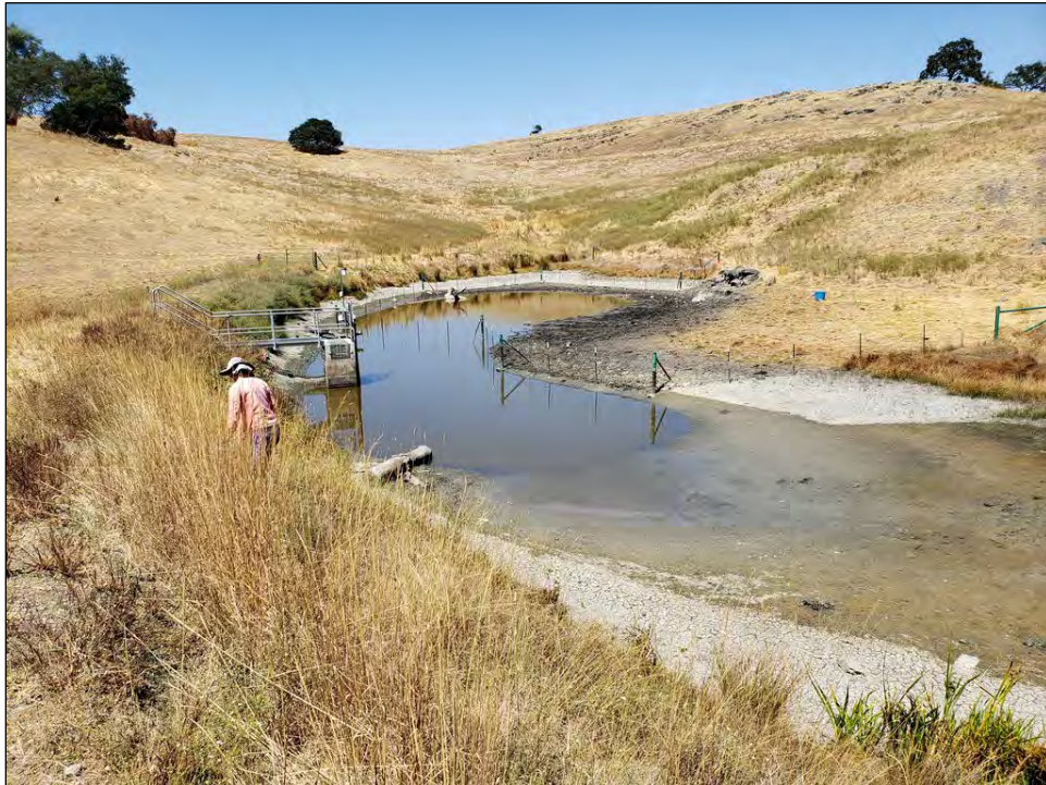
Photo 16. Year 3 Conditions at Photo Point 7a during Vegetation Monitoring at the Pond Mitigation Site (August 13, 2019)
