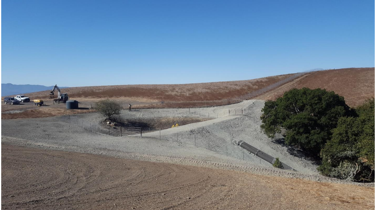
Photo 17. Post-Construction Photo Monitoring Point CR4_PPT1 (November 14, 2019)
