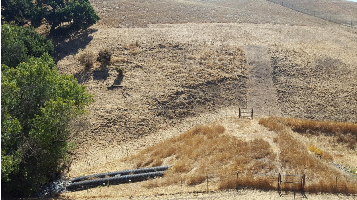
Photo 39. Year 1 Conditions at Photo Monitoring Point CR1_PPT2_2 (August 5, 2020)
