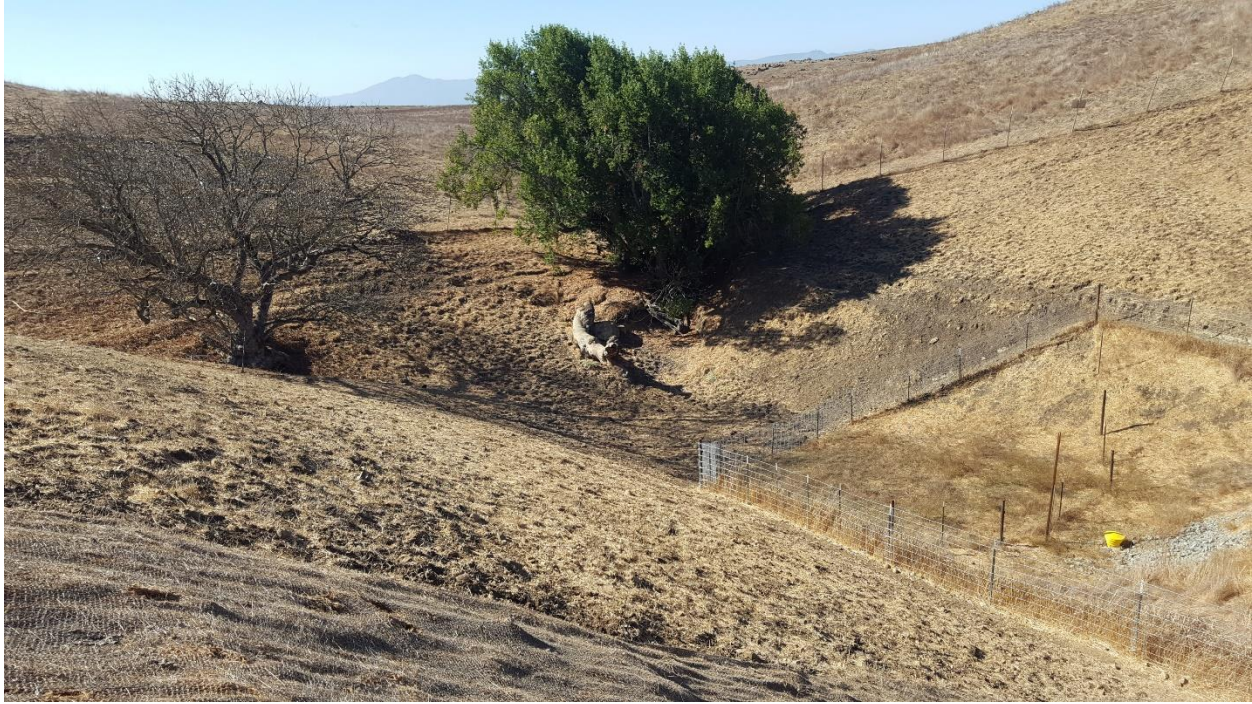
Photo 50. Year 1 Conditions at Photo Monitoring Point CR1_PPT3_1 (October 23, 2020)
