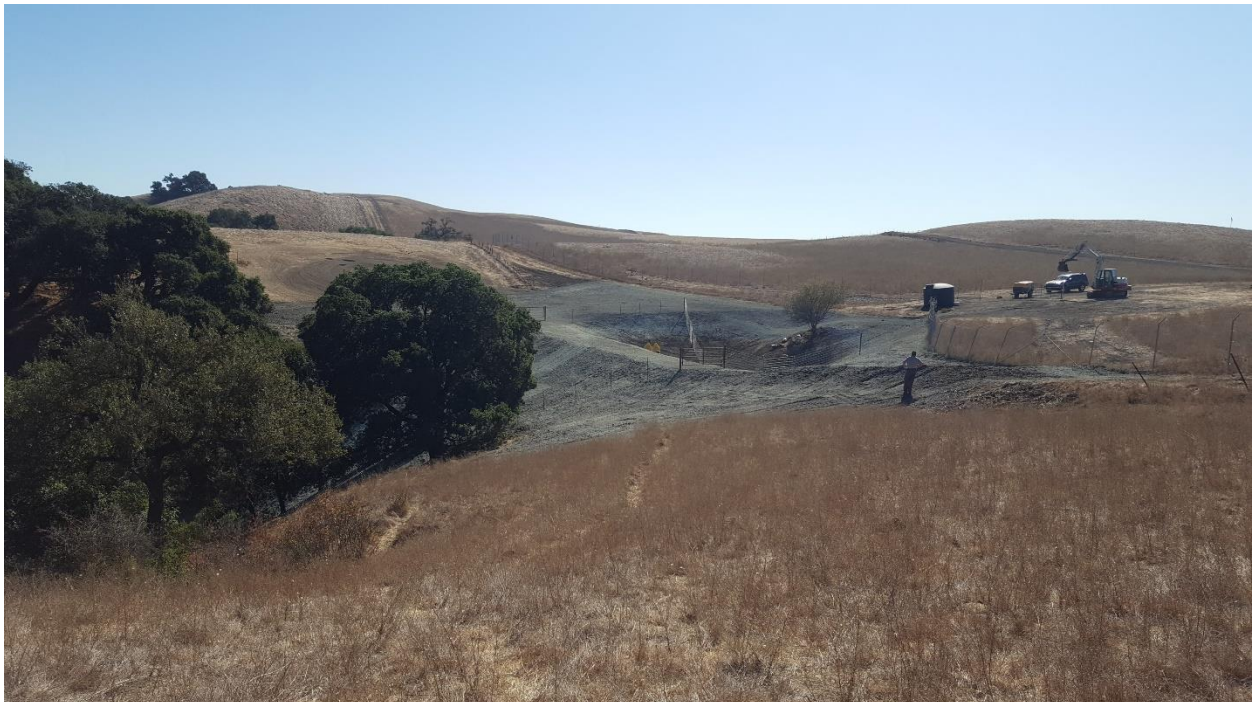
Photo 18. Post-Construction Photo Monitoring Point CR4_PPT2 (November 14, 2019)
