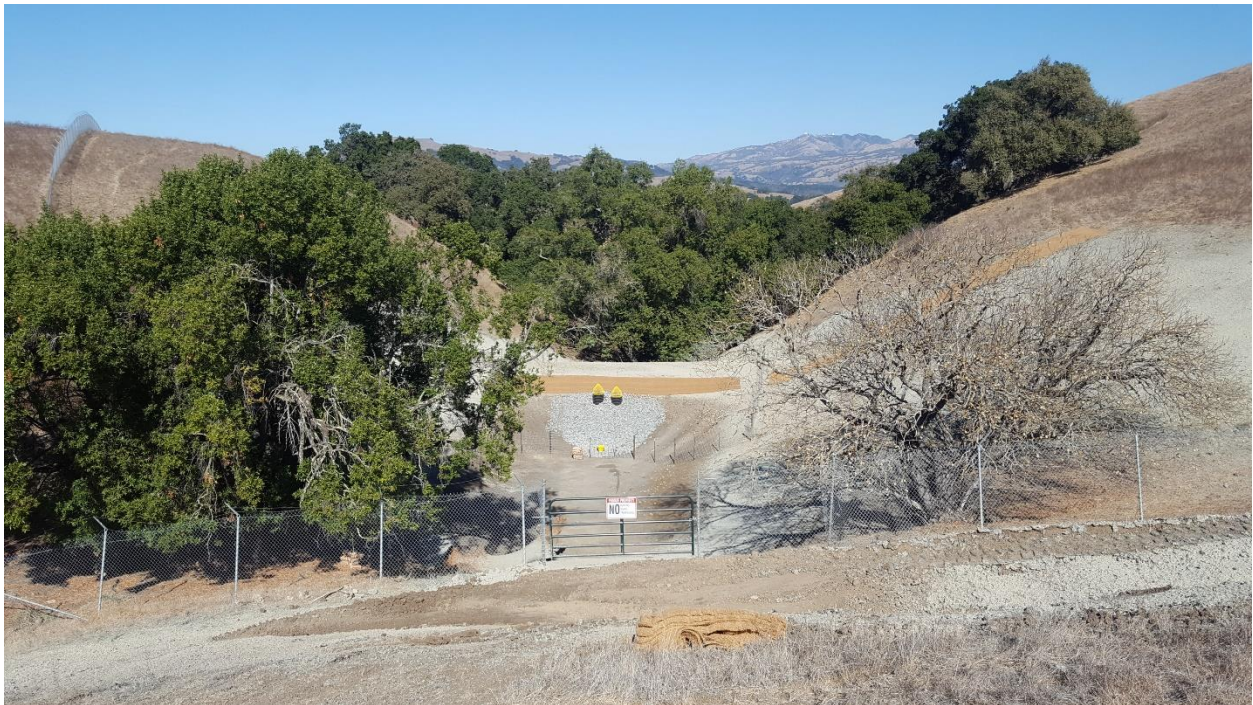
Photo 10. Post-Construction Photo Monitoring Point CR1_PPT1 (November 14, 2019)
