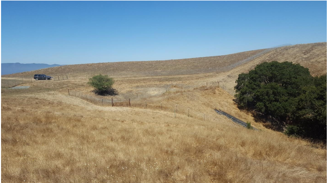
Photo 44. Year 1 Conditions at Photo Monitoring Point CR4_PPT1 (August 5, 2020)
