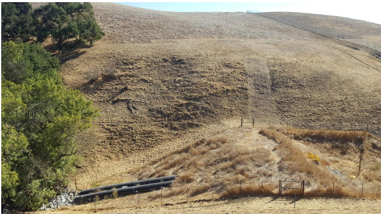
Photo 48. Year 1 Conditions at Photo Monitoring Point CR1_PPT2_2 (October 23, 2020)
