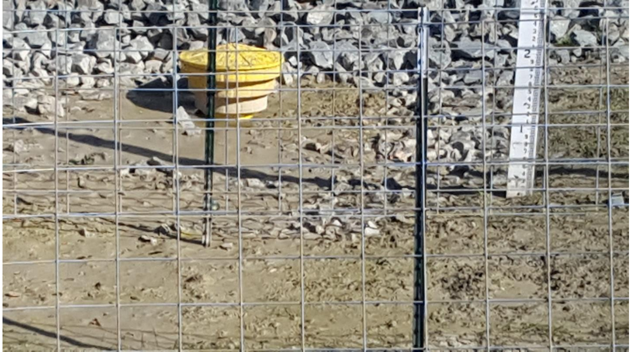
Photo 59. Completely Dry Pond Bed at CR4 (February 17, 2020)
