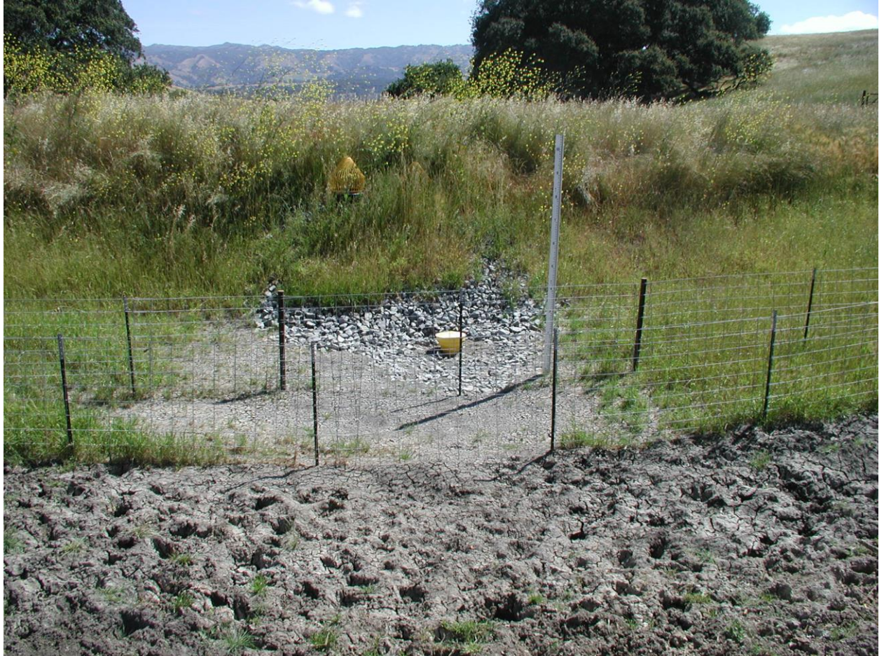
Photo 61. Completely Dry Pond Bed at CR4 (May 16, 2020)
