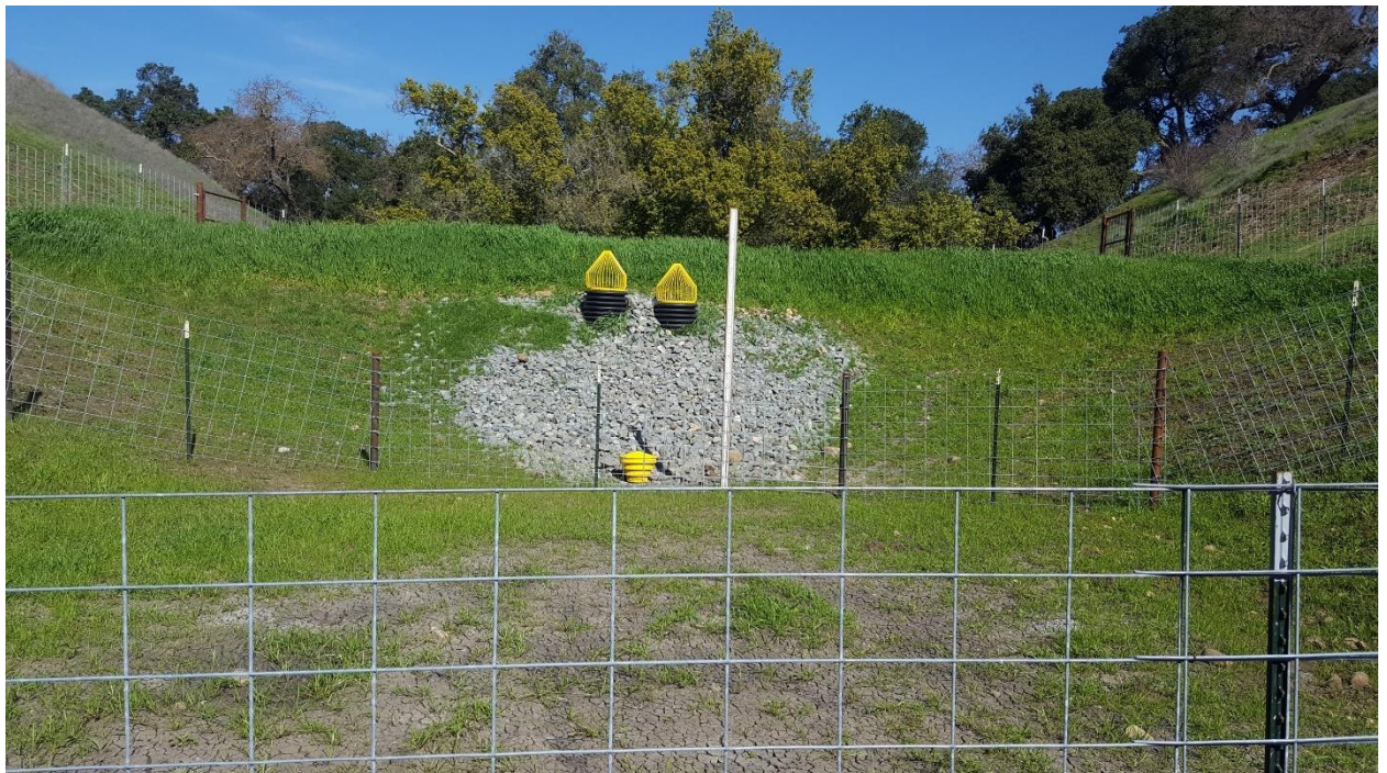
Photo 56. Completely Dry Pond Bed at CR1 (February 17, 2020)
