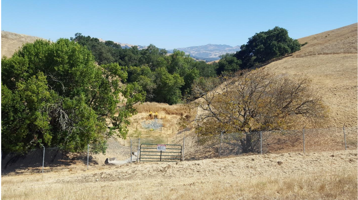
Photo 37. Year 1 Conditions at Photo Monitoring Point CR1_PPT1 (August 5, 2020)
