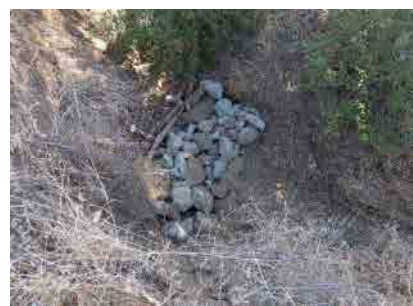
6 STAKED DEBRIS JAM (HANDWORK ONLY) SCALE: NTS
