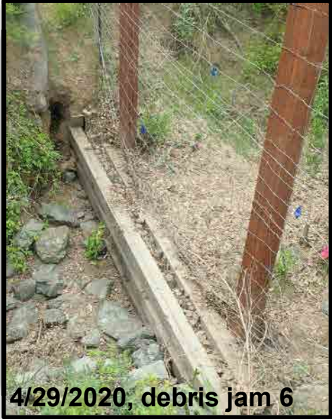
Figure 16. Staked debris jams at ID02-01, April 29, 2020, San Felipe Creek Restoration Project, Joseph D. Grant Park, Santa Clara County, California.
