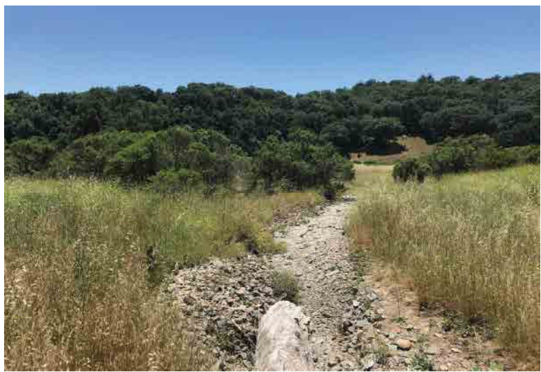
Photo 32a: Southwest - ID01 - 06/19/19
