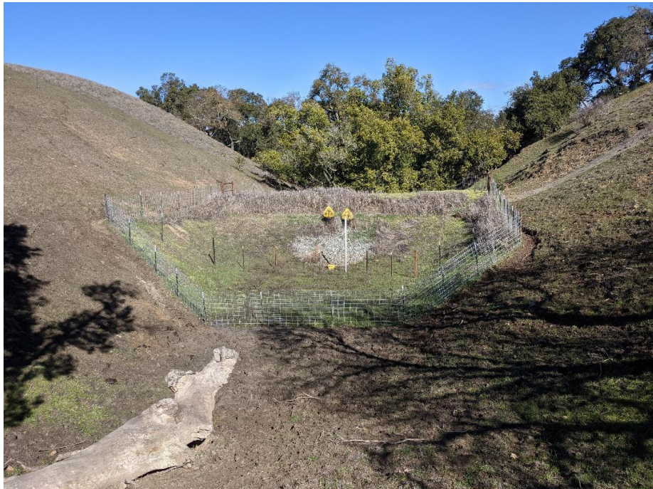
Photo 29. Completely Dry Pond Bed at CR1 (February 1, 2021)
