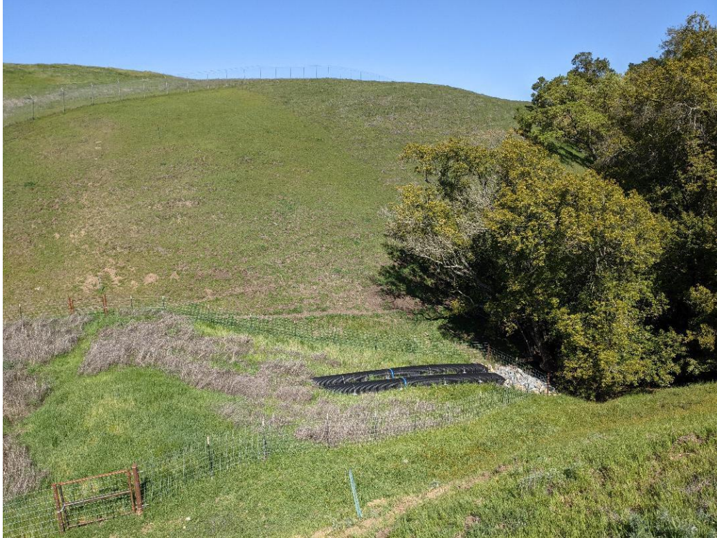
Photo 18. Year 2 Conditions at Photo Monitoring Point CR1_PPT3_2 (April 8, 2021)
