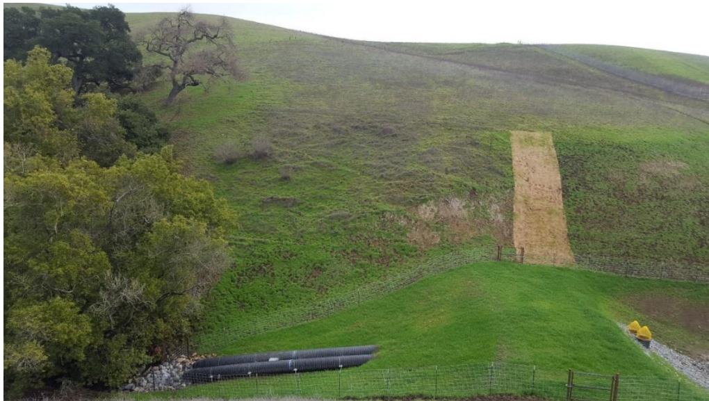
Photo 8. Year 1 Conditions at Photo Monitoring Point CR1_PPT2_2 (January 28, 2020)
