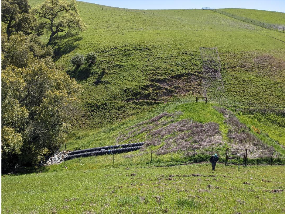
Photo 9. Year 2 Conditions at Photo Monitoring Point CR1_PPT2_2 (April 8, 2021)
