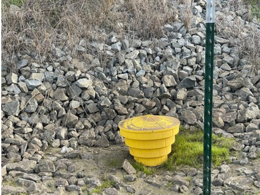
Photo 32. No water at CR4 due to open drain valve (photo provided by SCVHA, February 10, 2021)
