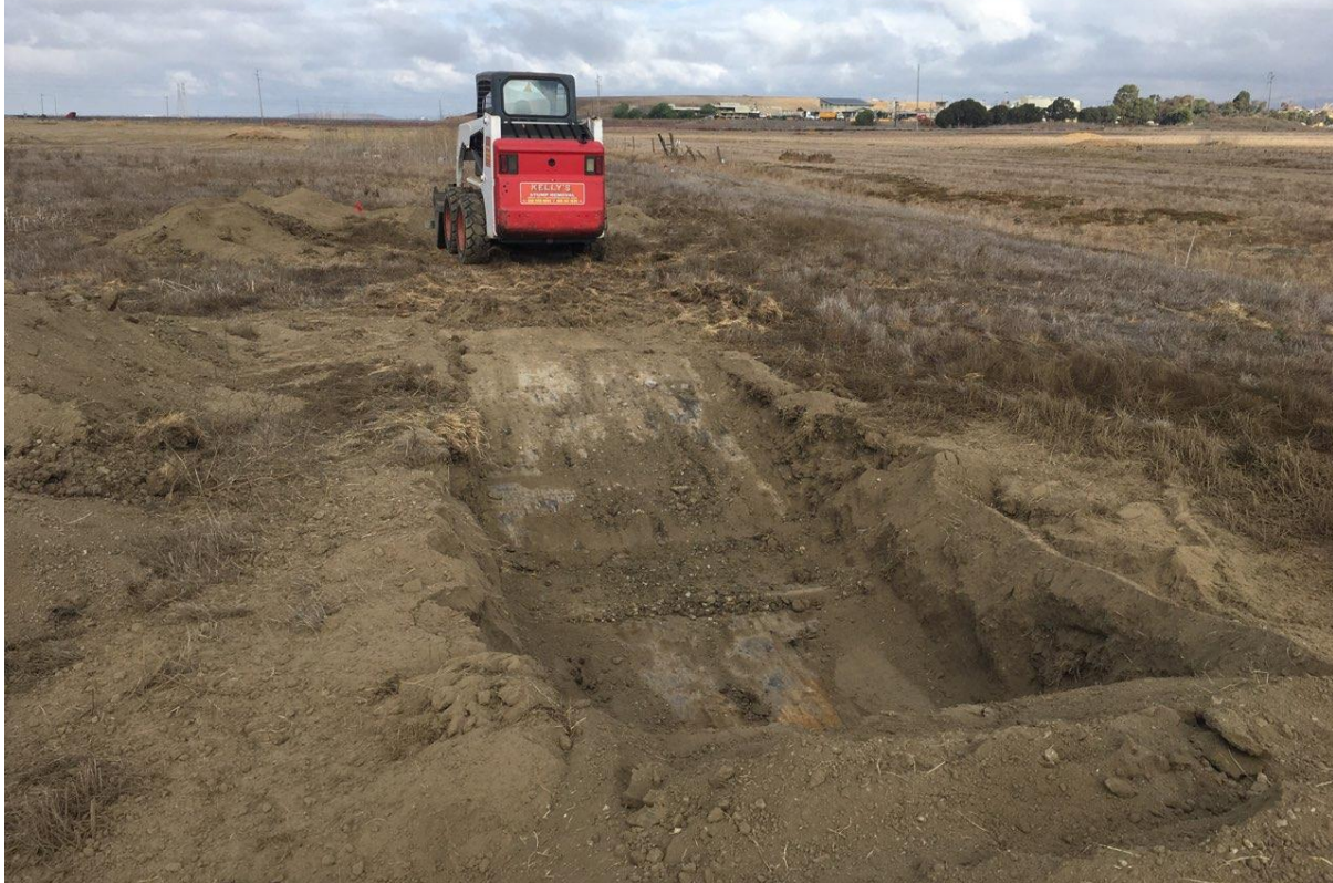
Figure 11. Excavation for installing an artificial burrow complex. (Photograph taken in November 2020)
