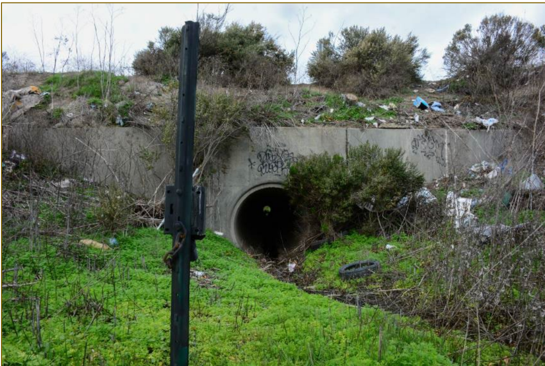
Figure 27. View of westbound opening. Facing north.
