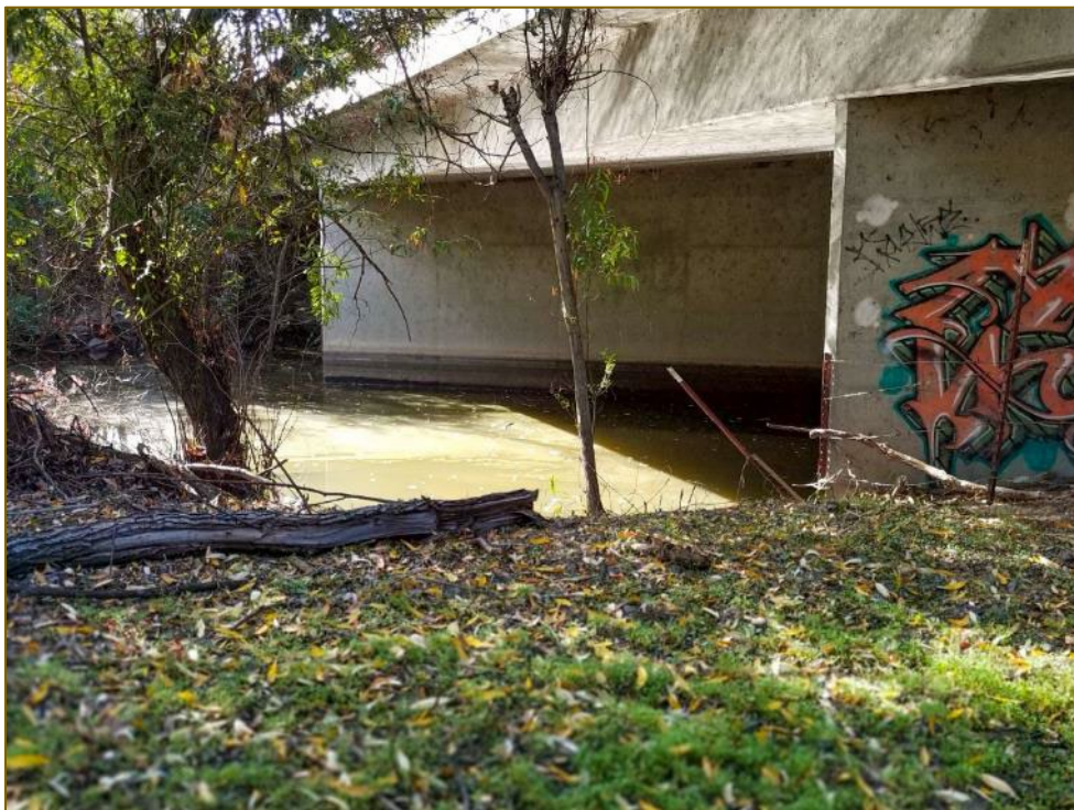
Figure 4. View of eastbound opening showing water level, and fencing. Facing west.
