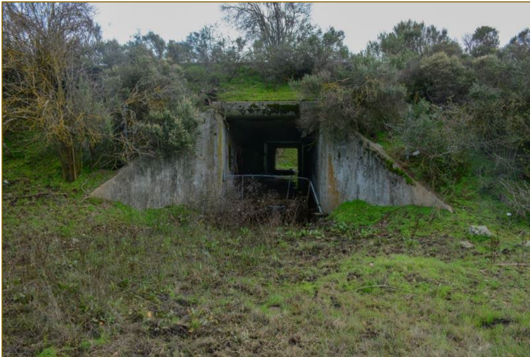
Figure 25. West bound opening of culvert PM 34.64. Facing north.
