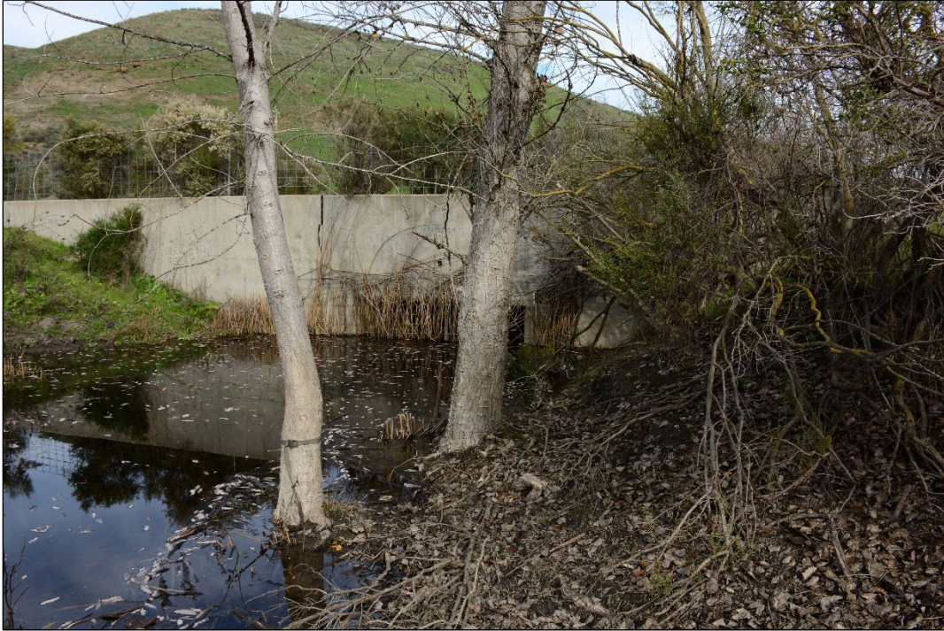
Figure 6. Laguna Seca culvert at Santa Teresa Boulevard culvert, west side on 1/13/2021.
