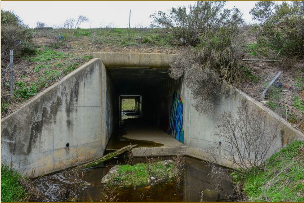
Figure 26. Culvert 34.64 eastbound opening. Facing north.
