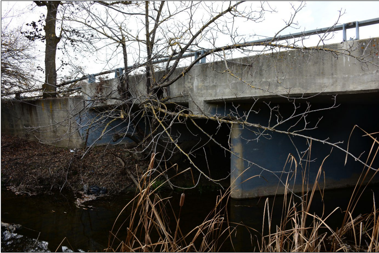
Figure 12: Bailey Bridge at Fisher Creek on 1/13/2022.
