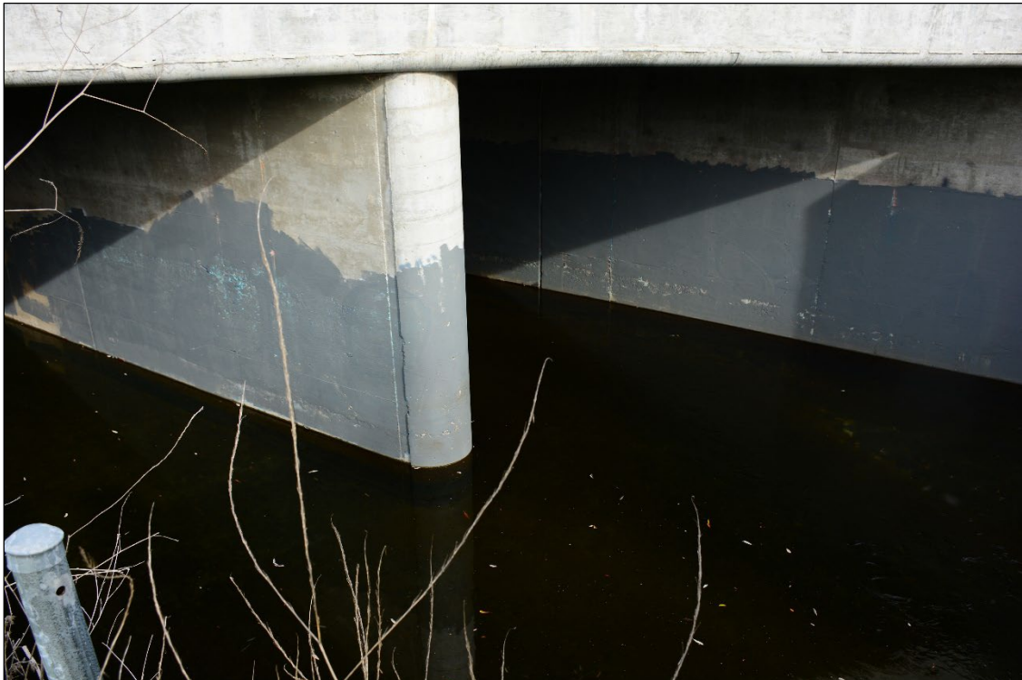
Figure 5. Santa Teresa Boulevard culvert, west side on 1/13/2021.
