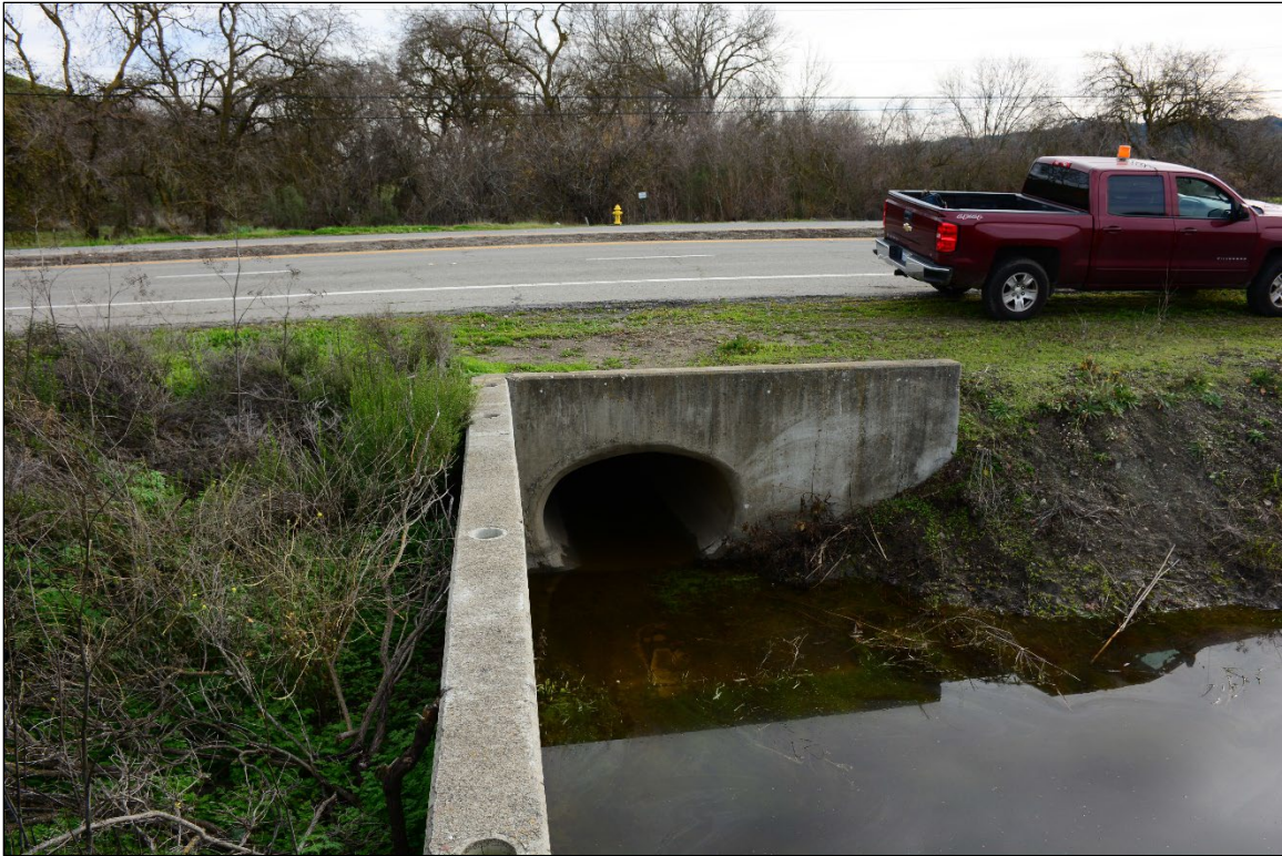
Figure 4. Bailey culvert, north side on 1/13/2021.
