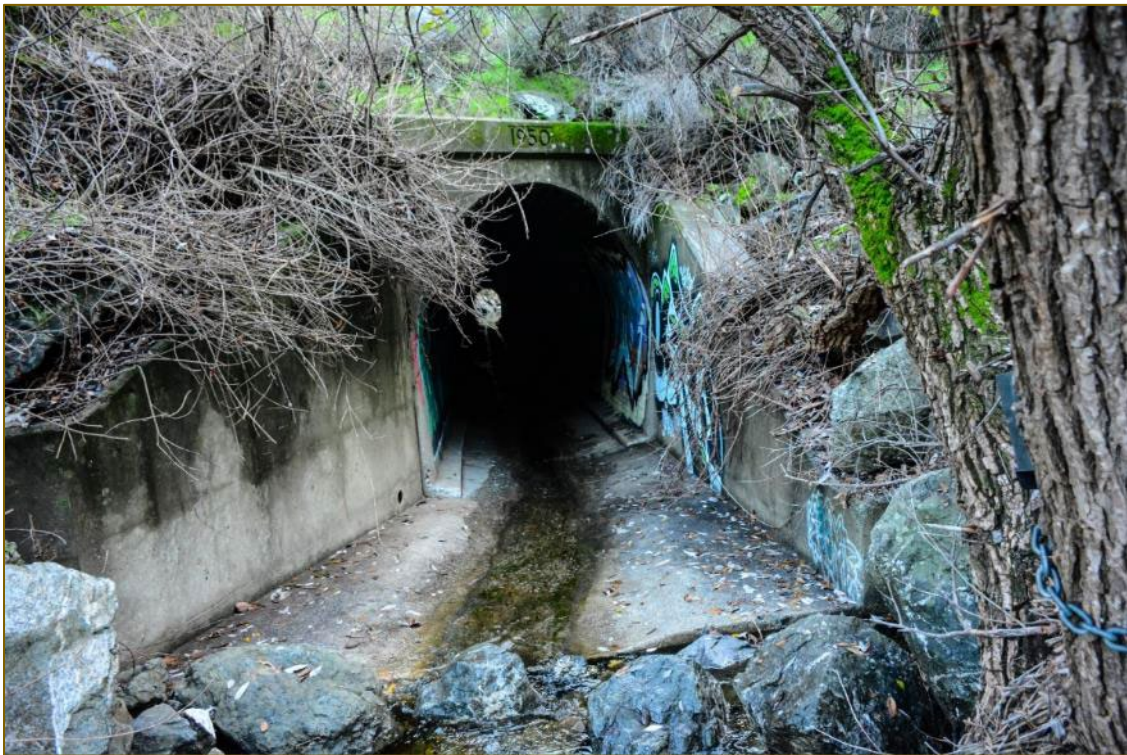
Figure 11. Westbound opening of culvert PM 32.61. Facing south.
