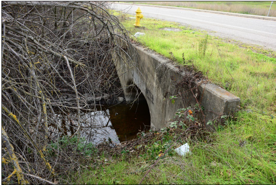
Figure 2. Bailey culvert, south side on 1/13/2021.
