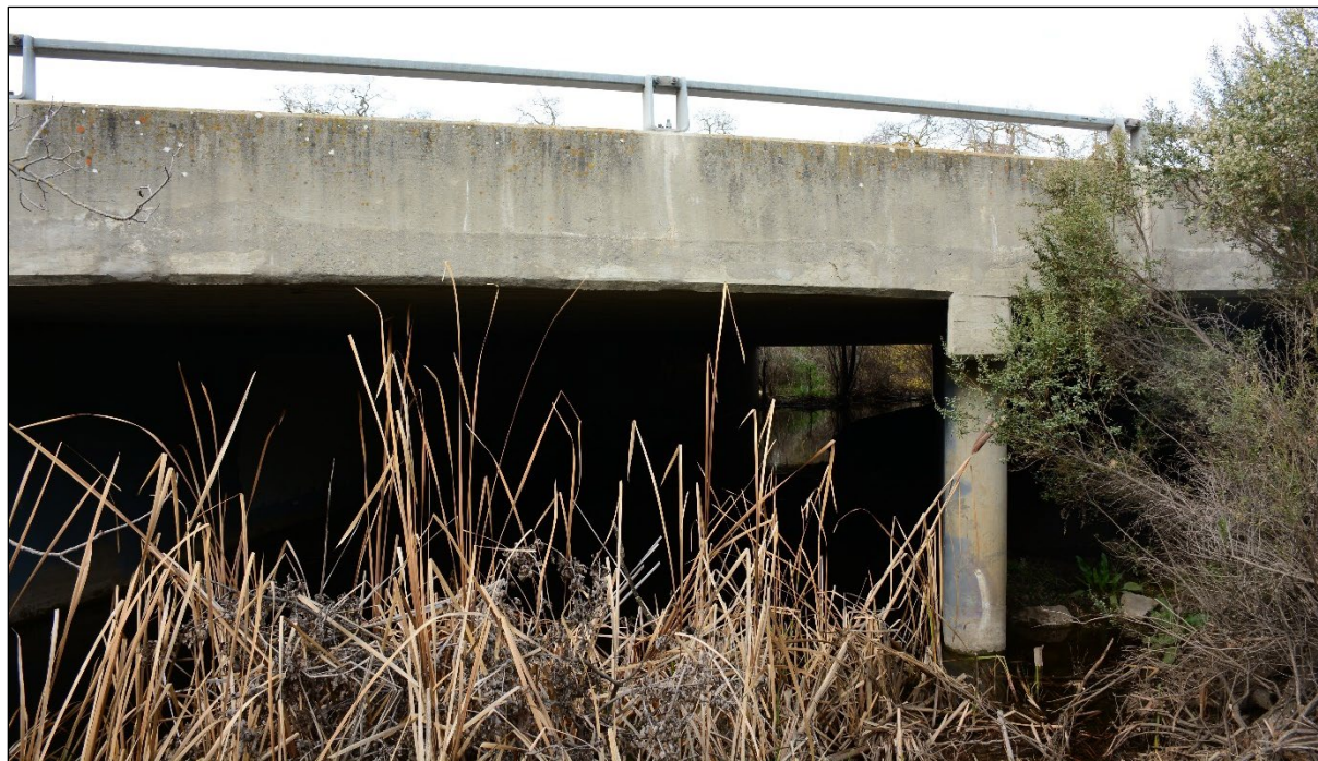
Figure 13: Bailey Bridge at Fisher Creek on 1/13/2022.
