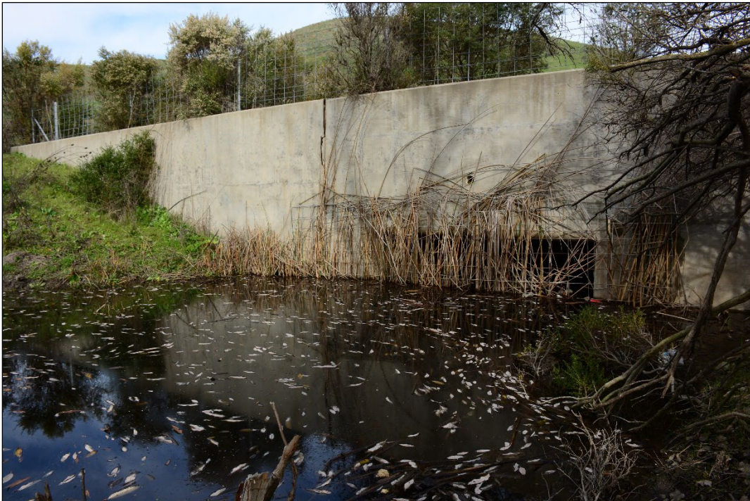
Figure 7. Laguna Seca culvert at Santa Teresa Boulevard culvert, west side on 1/13/2021.
