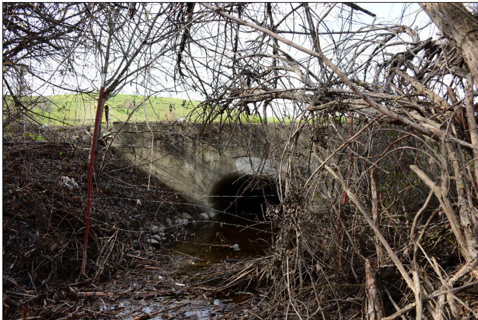
Figure 3. Bailey culvert, south side on 1/13/2021.
