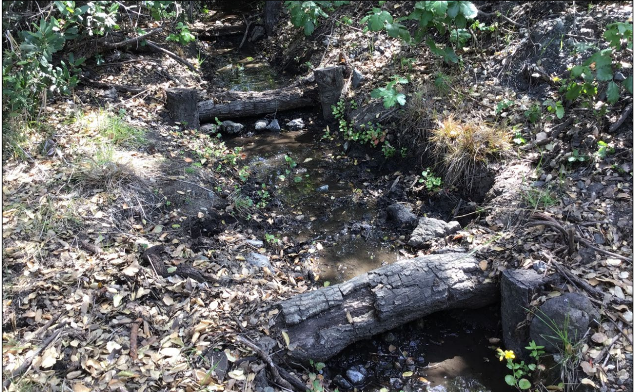
Photo 36. Year 6 Conditions at Photo Point 15 during Vegetation Monitoring, with a Log Debris Jam Installed in the Seep Collection Area (April 6, 2022)
