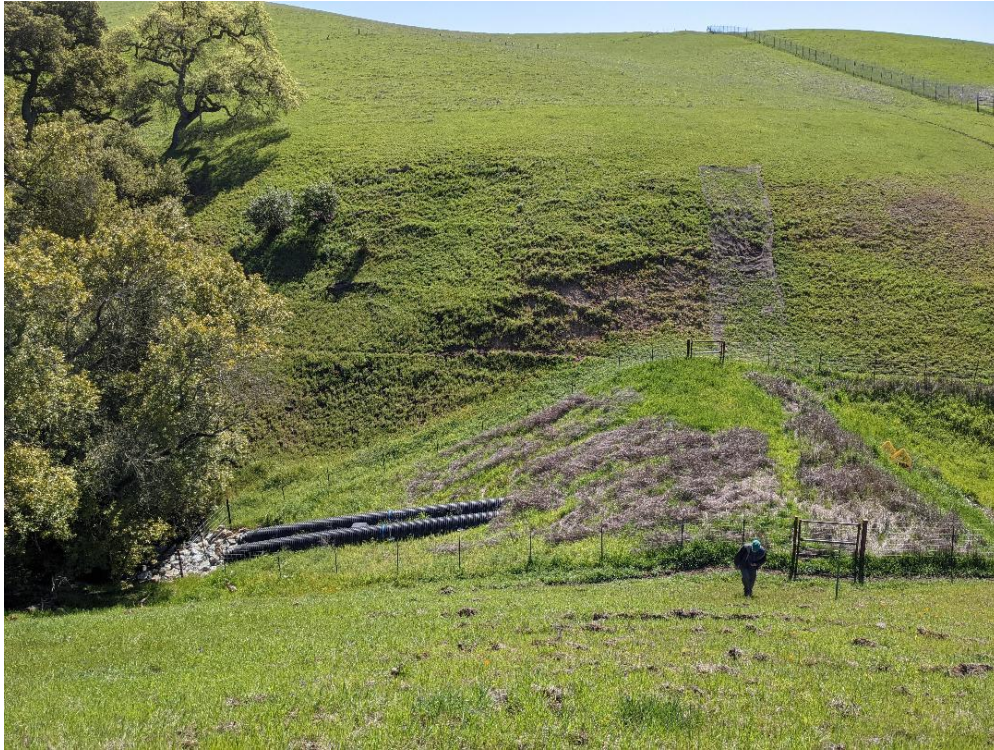
Photo 11. Year 2 Conditions at Photo Monitoring Point CR1_PPT2_2 (April 8, 2021)
