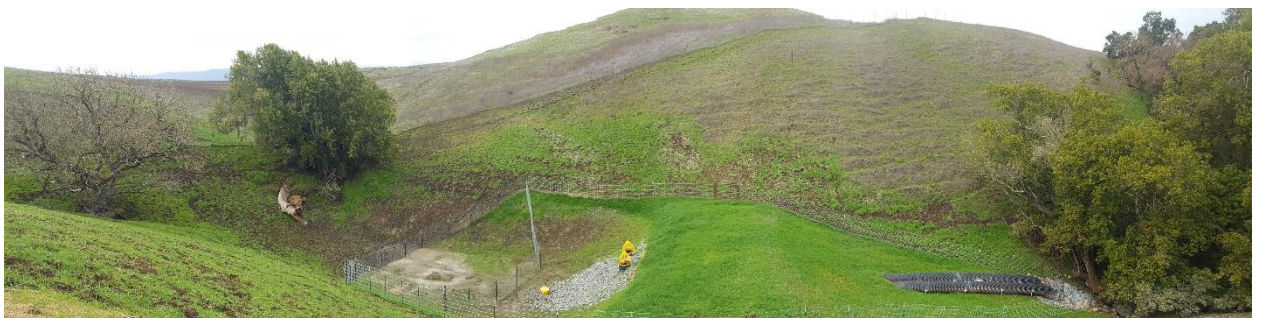
Photo 26. Year 1 Conditions at Photo Monitoring Point CR1_PPT3_3 (January 28, 2020)
