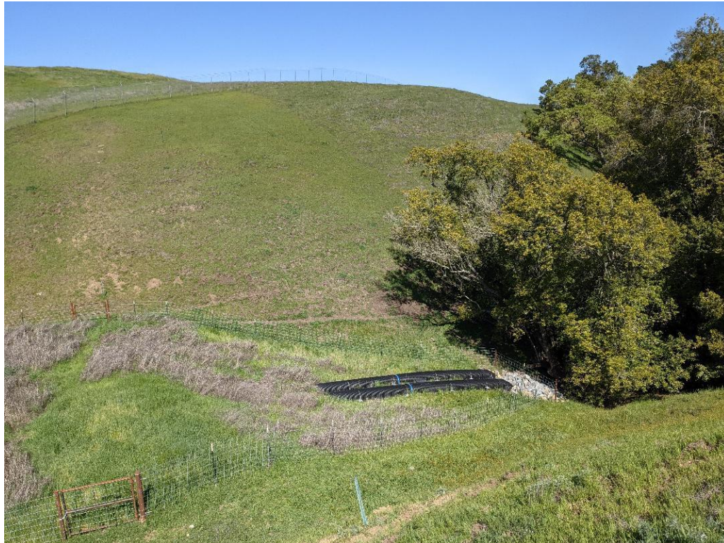
Photo 23. Year 2 Conditions at Photo Monitoring Point CR1_PPT3_2 (April 8, 2021)
