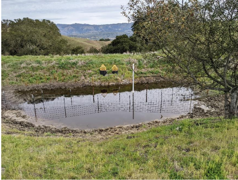
Photo 43. 2.1-ft of water at CR4 (March 3, 2022)
