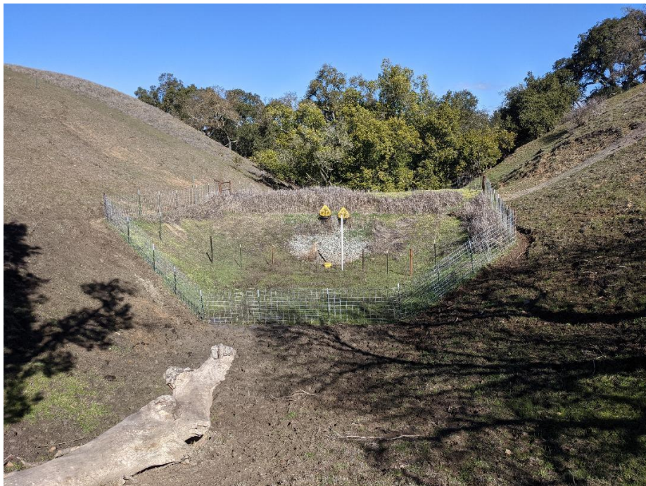
Photo 38. Completely Dry Pond Bed at CR1 (February 1, 2021)
