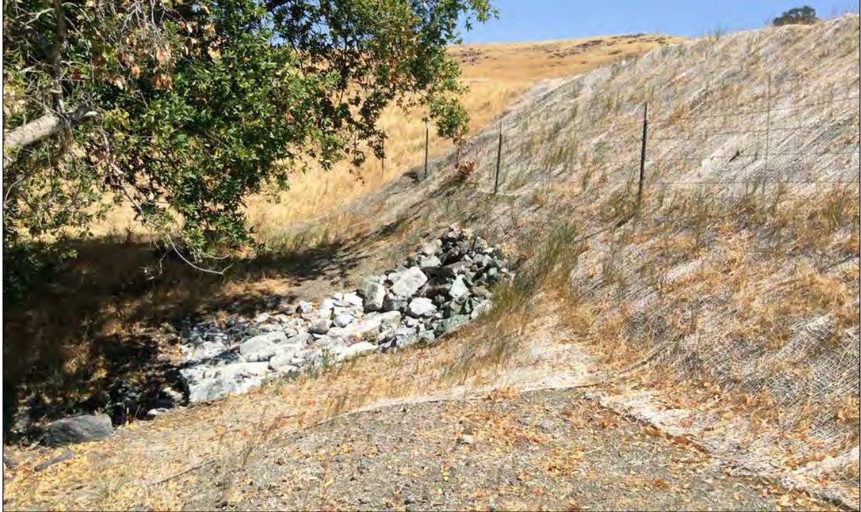
Photo 9. Year 1 Conditions at Photo Point 8 during Vegetation Monitoring at the Pond Mitigation Site (August 8, 2017)
