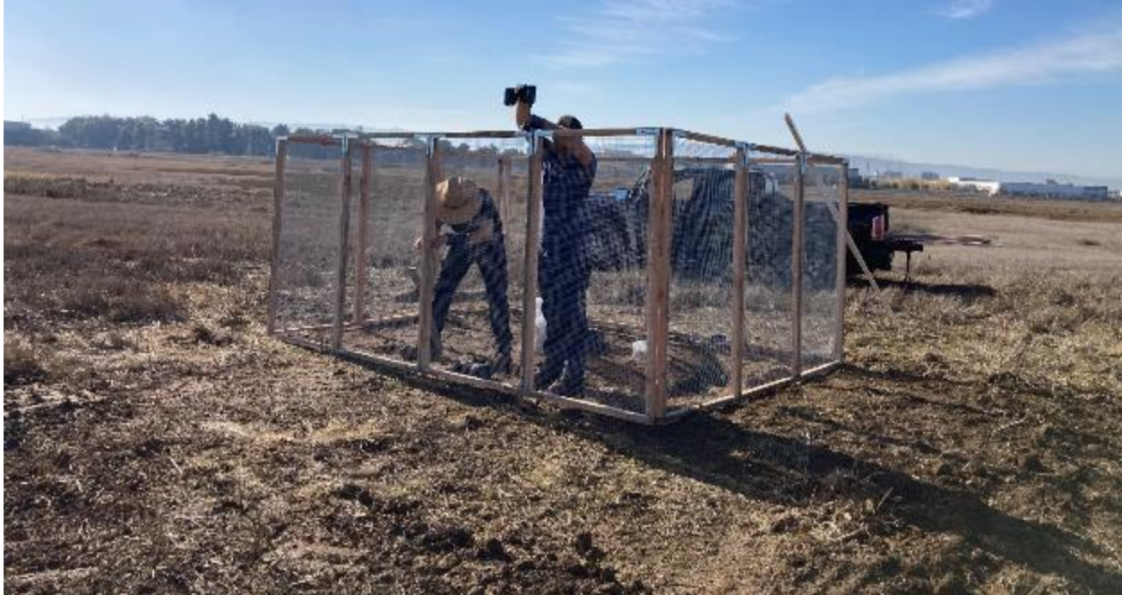
Figure 3. Construction of hacking enclosures for the soft-release of breeding pairs of burrowing owls as part of the Juvenile Burrowing Owl Overwintering Project.
