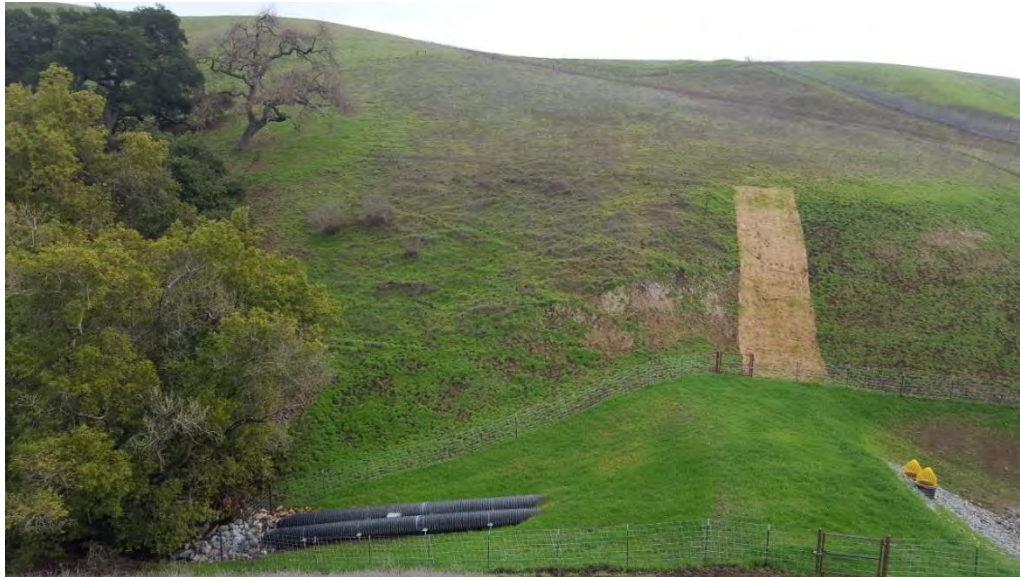
Photo 12. Year 1 Conditions at Photo Monitoring Point CR1_PPT2_2 (January 28, 2020)
