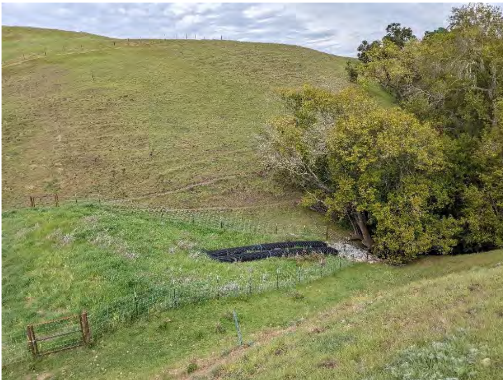
Photo 29. Year 3 Conditions at Photo Monitoring Point CR1_PPT3_2 (March 3, 2022)
