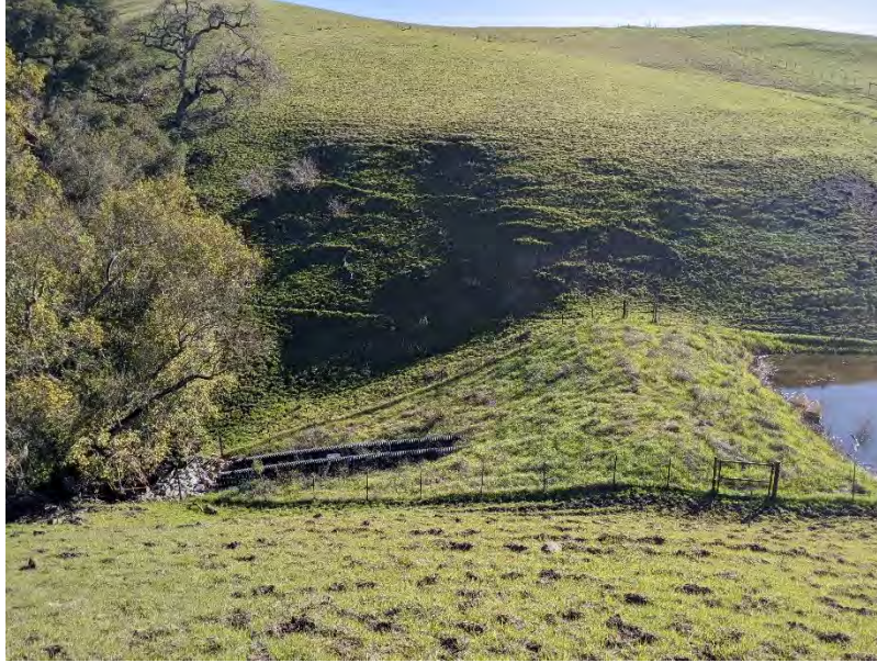
Photo 15. Year 4 Conditions at Photo Monitoring Point CR1_PPT2_2 (January 30, 2023)
