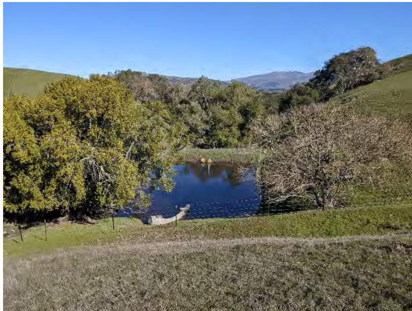
Photo 42. CR1 filled and flowing into overflow pipes with >12-inches of rainfall in November – January (January 30, 2023).
