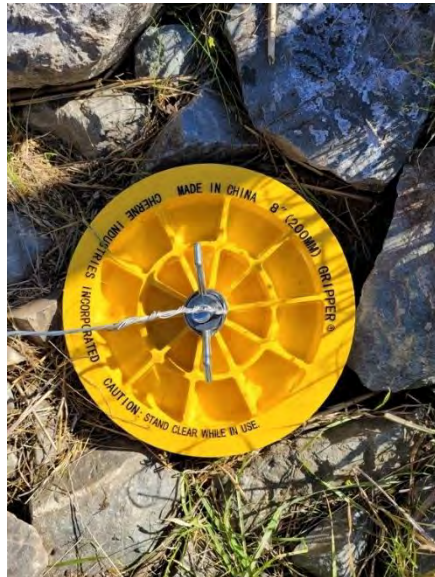
Photo 33. Removeable caps, added to the quick drain pipes to prevent leakage (photo provided by SCVHA, November 30, 2021)
