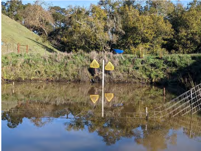
Photo 39. 4.6 feet of water at CR1 (January 14, 2022)
