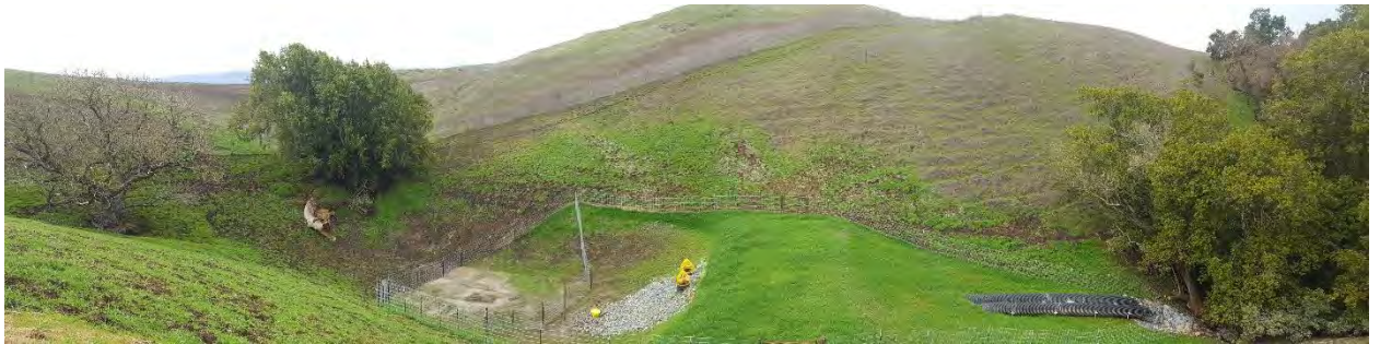
Photo 32. Year 1 Conditions at Photo Monitoring Point CR1_PPT3_3 (January 28, 2020)
