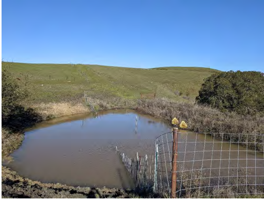
Photo 44. Pond remains filled with 4.9 ft of water (April 19, 2023)
