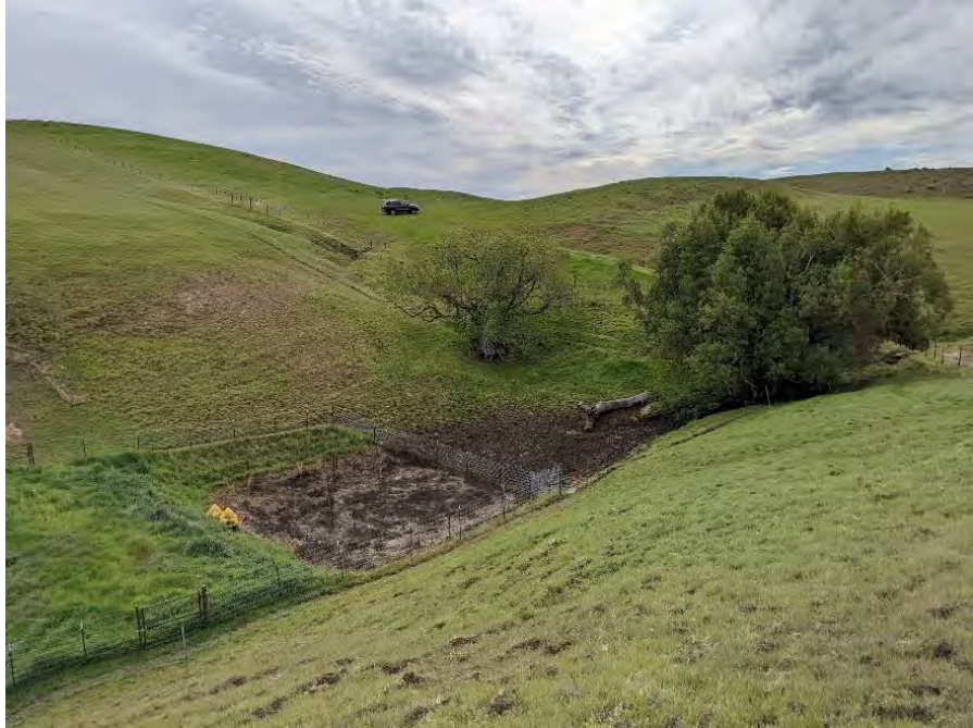
Photo 9. Year 3 Conditions at Photo Monitoring Point CR1_PPT2_1 (March 3, 2022)
