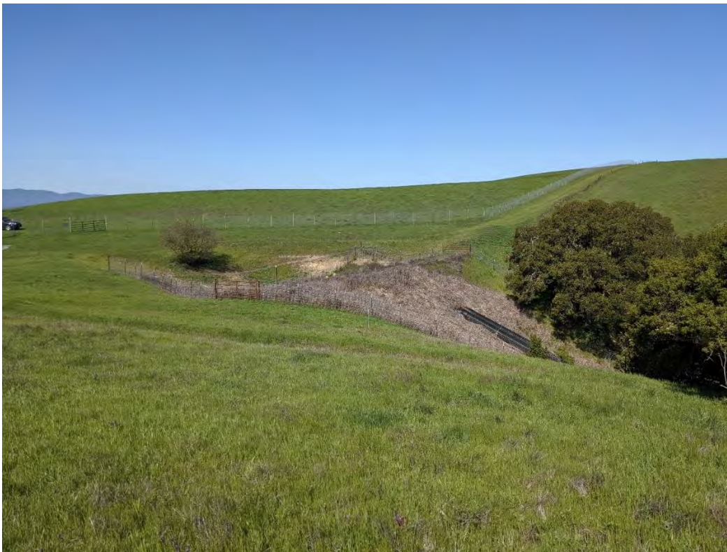
Photo 38. Year 2 Conditions at Photo Monitoring Point CR4_PPT1 (April 8, 2021)
