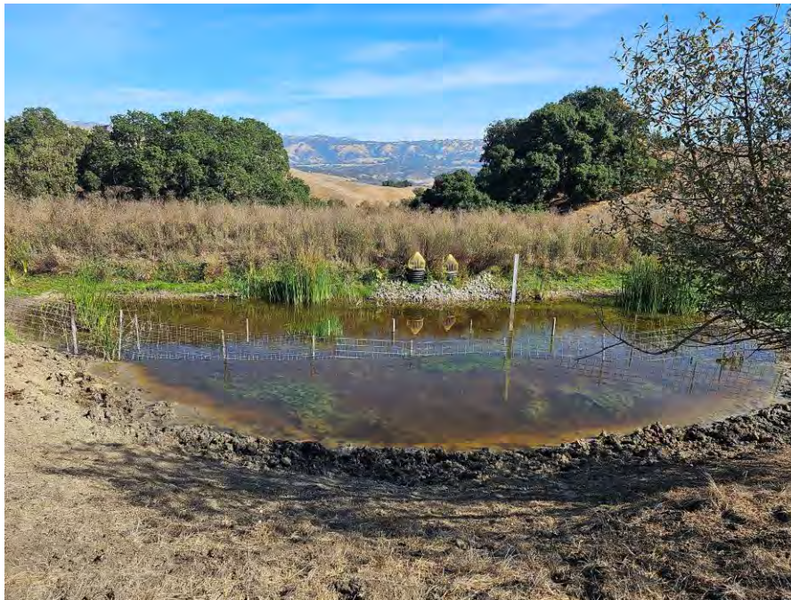
Photo 45. Pond did not dry during the summer months and retained 3.1 ft of water (November 2, 2023)
