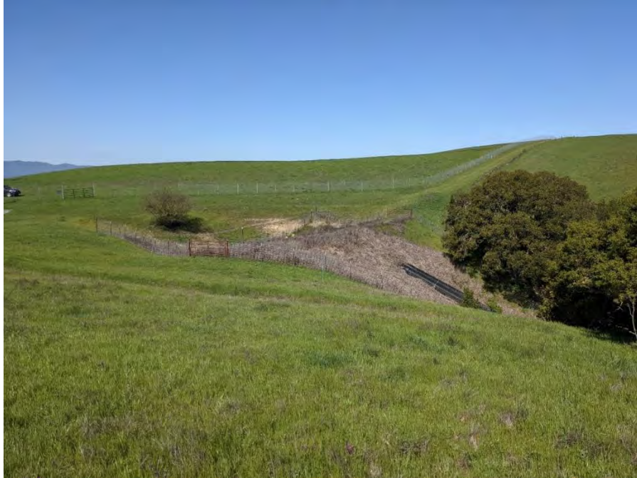
Photo 43. Year 2 Conditions at Photo Monitoring Point CR4_PPT2 (April 8, 2021)
