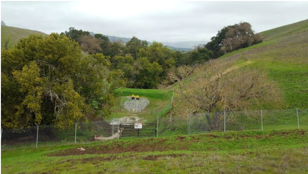
Photo 2. Year 1 Conditions at Photo Monitoring Point CR1_PPT1 (January 28, 2020)
