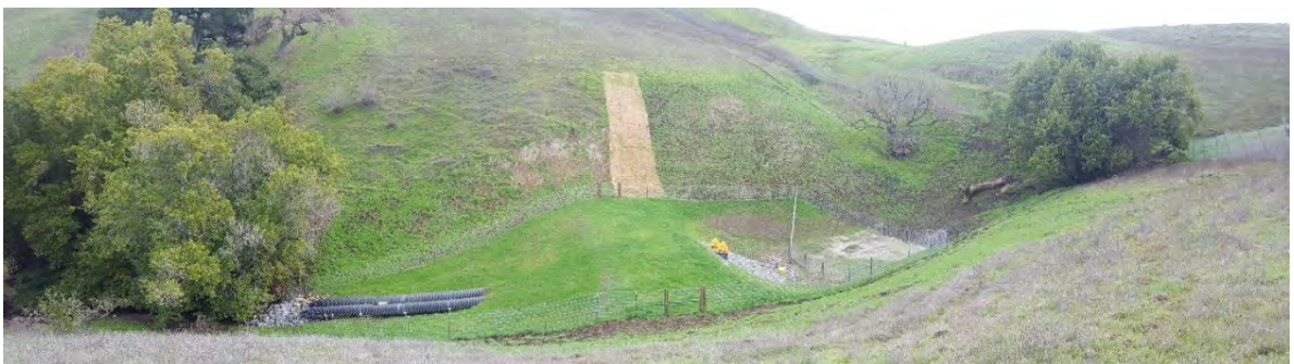
Photo 17. Year 1 Conditions at Photo Monitoring Point CR1_PPT2_3 (January 28, 2020)
