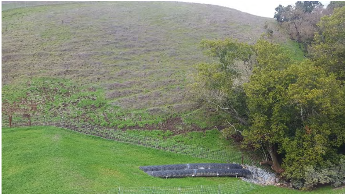
Photo 27. Year 1 Conditions at Photo Monitoring Point CR1_PPT3_2 (January 28, 2020)
