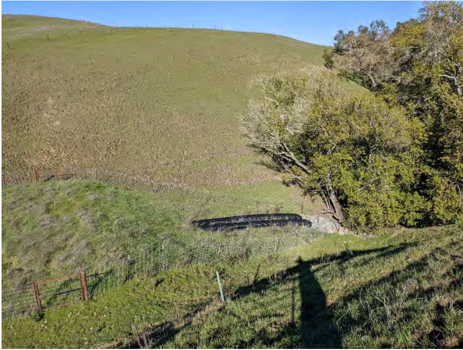
Photo 30. Year 4 Conditions at Photo Monitoring Point CR1_PPT3_2 (January 30, 2023)
