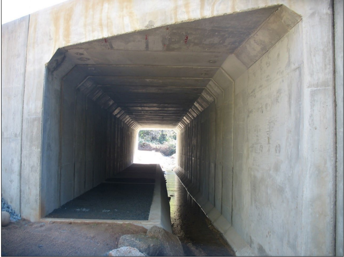
Figure 111. Culvert retrofit on SR-89 by Ken Russo, Senior Environmental Planner, Branch Chief Unit M5, Resource Biologist, Caltrans, District 3.
