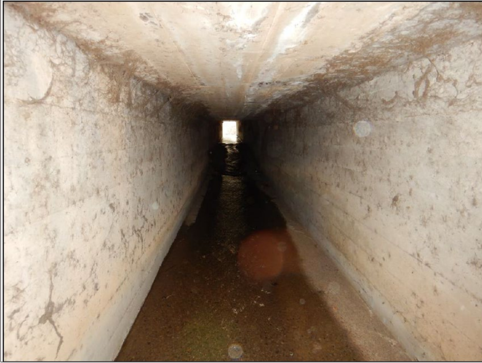
Figure 50. View from within eastbound opening of culvert C12 PM 27.24.
