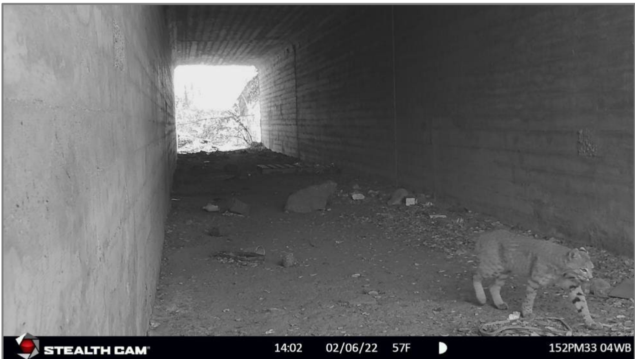
Figure 80. A bobcat crossing through SR-152 culvert C20 PM 33.04 on February 6, 2022.
