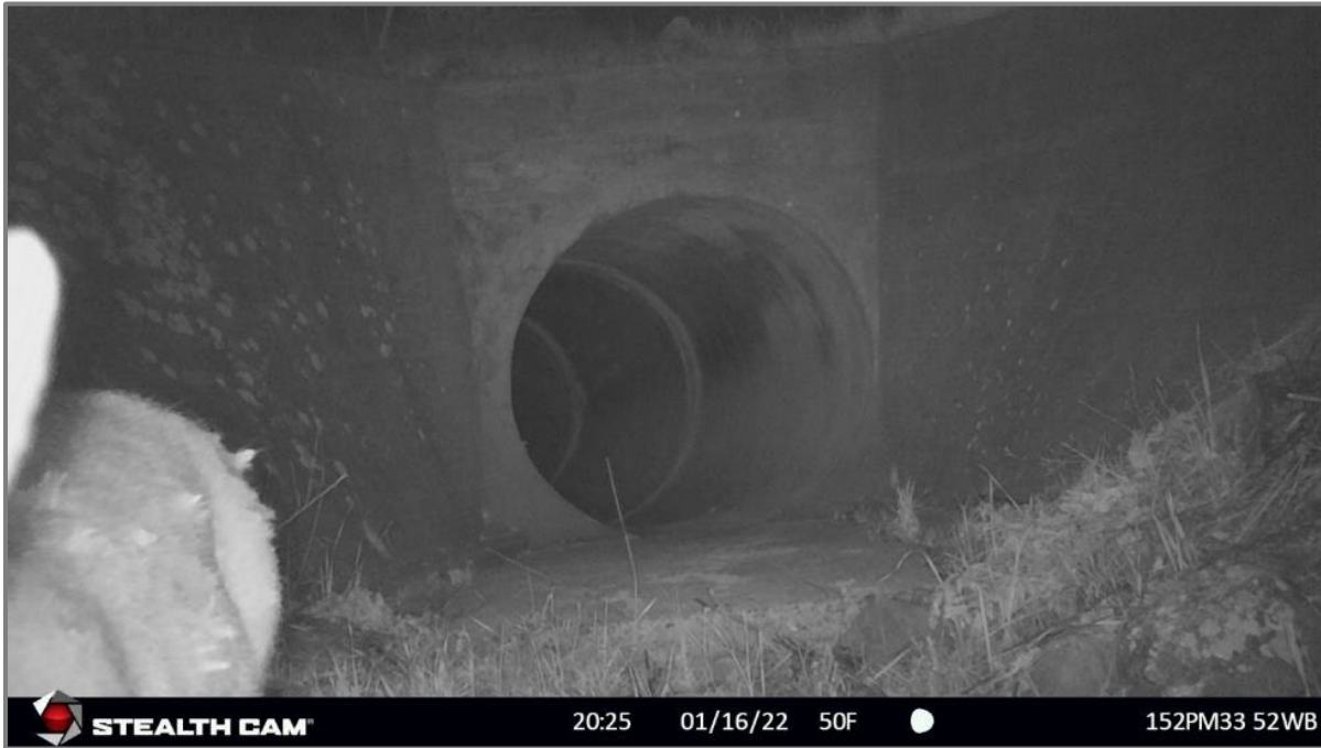
Figure 83. Deer turning away from SR-152 culvert C21 PM 33.52 on January 16, 2022.
