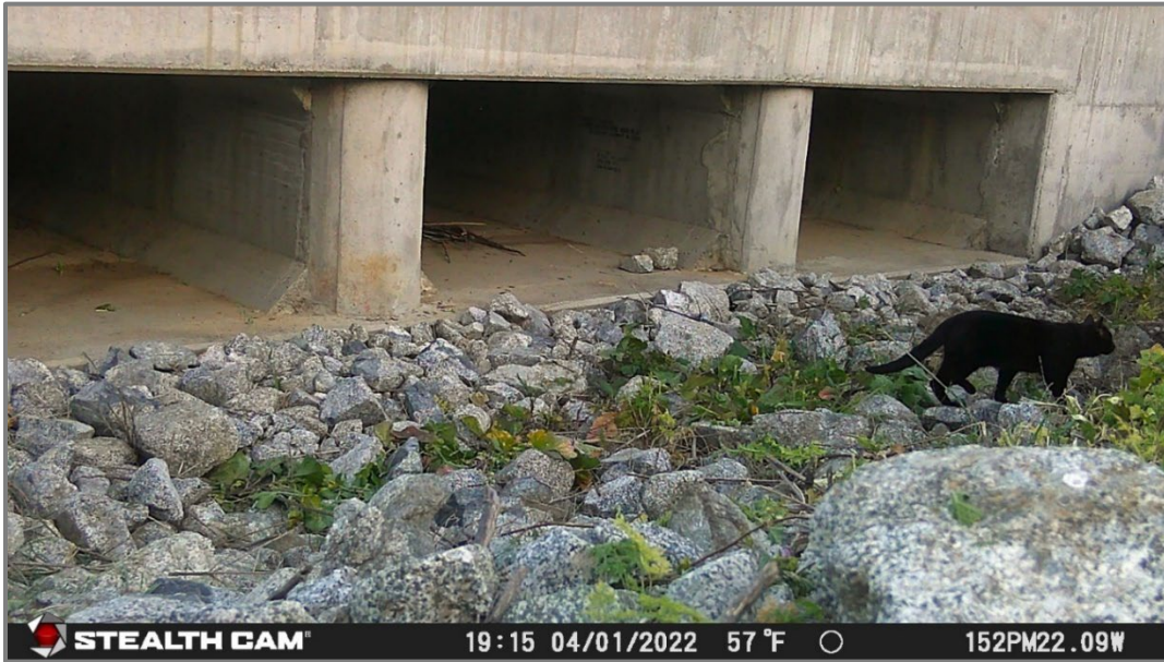
Figure 24. Domestic cat at culvert C7 PM 22.09 on April 1, 2022.
