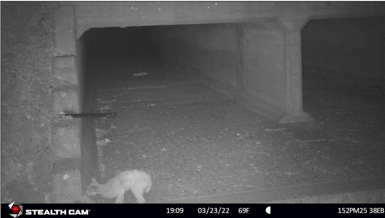
Figure 92. Bobcat with mange at the Killdeer Creek Bridge/Elephant Head Creek culvert.
