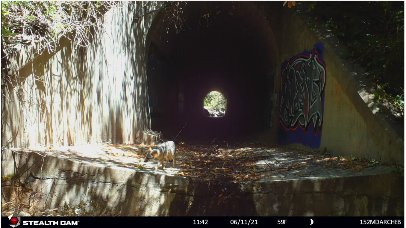
Figure 74. A gray fox crossing through culvert C17 PM 32.3.
