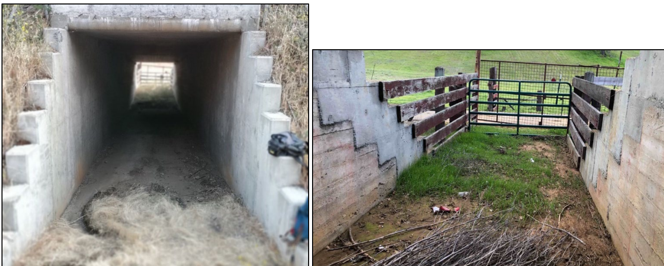
Figure 14. C3 large box culvert. Gate visible at opposite opening.
