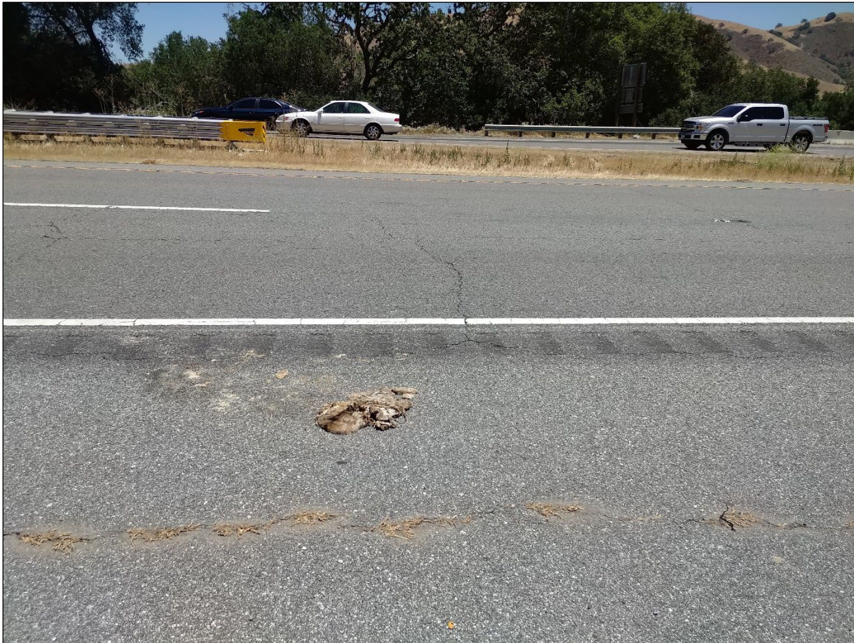
Figure 111. Coyote found hit on June 24, 2022, westbound lane by Walnut Ave. This is by the culvert where domestic dogs have been recorded chasing wildlife through the culvert.
