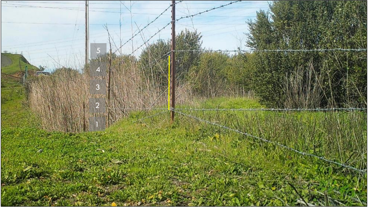
Figure 8. Five-strand barbed wire with a gap between the second and third strand from bottom.
