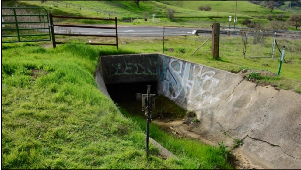
Figure 78. Coyote Alamitos Canal, northbound, on the west side of Tulare Hill.
