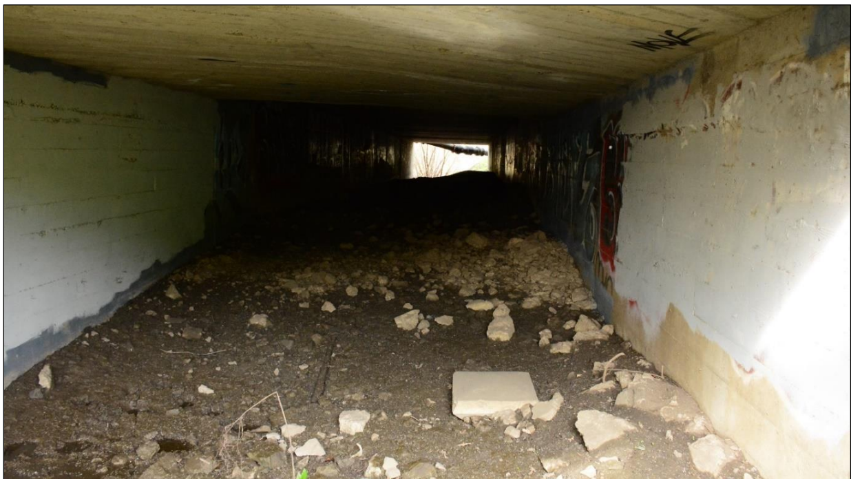
Figure 114. Bailey Bridge at Fisher Creek on 1/13/2022, eastern section of the bridge.
