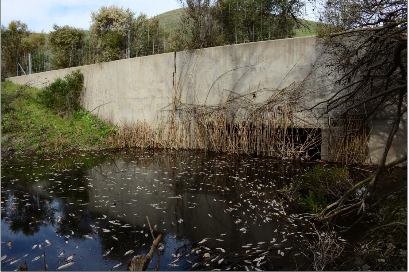
Figure 93. Laguna Seca culvert at Santa Teresa Boulevard culvert, west side on 1/14/2021.
