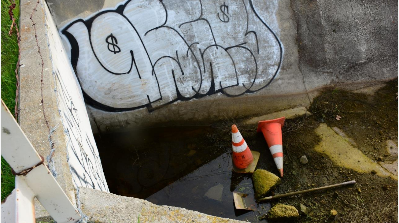
Figure 94. Coyote Alamitos Canal culvert, west side on 1/13/2021.
