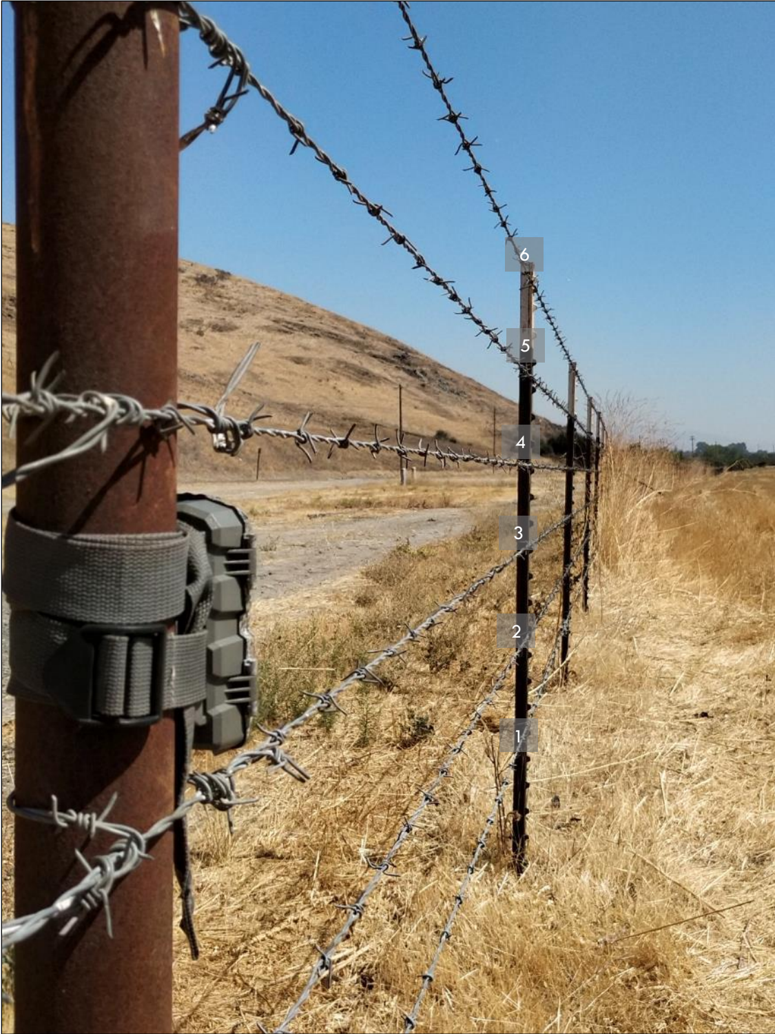
Figure 9. Six-strand barbed wire, fencing along the west side of Laguna Seca at Santa Teresa Blvd.
