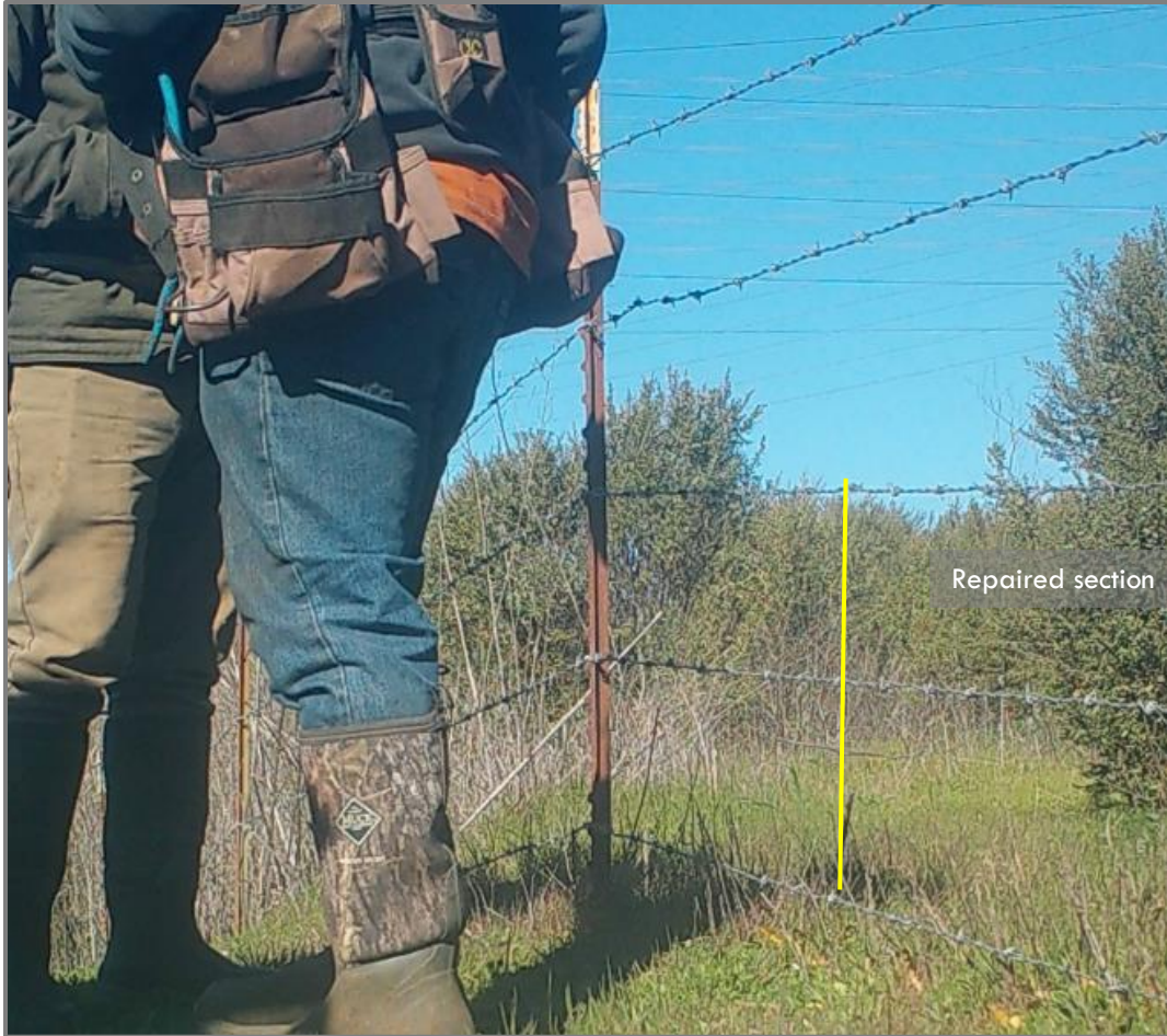
Figure 33. Two fence repair crewmembers fixing gap in five-strand barbed wire fence on 02/02/2022 at Santa Teresa Laguna Seca fence line camera site 2.
