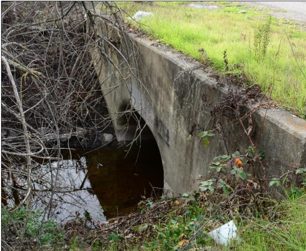
Figure 88. Bailey Ave. culvert south side on 1/14/2021.
