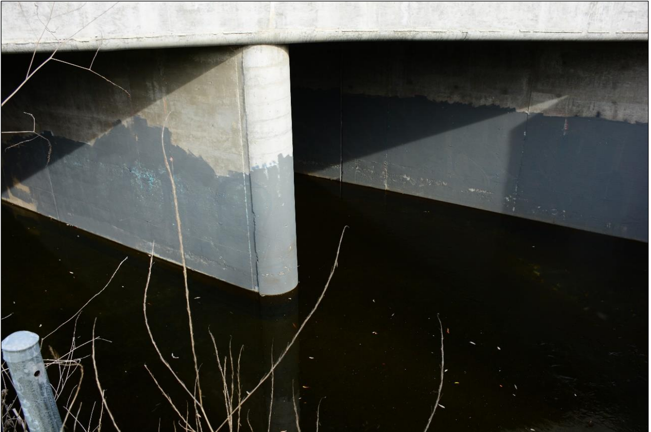
Figure 92. Santa Teresa Boulevard culvert, west side on 1/14/2021.
