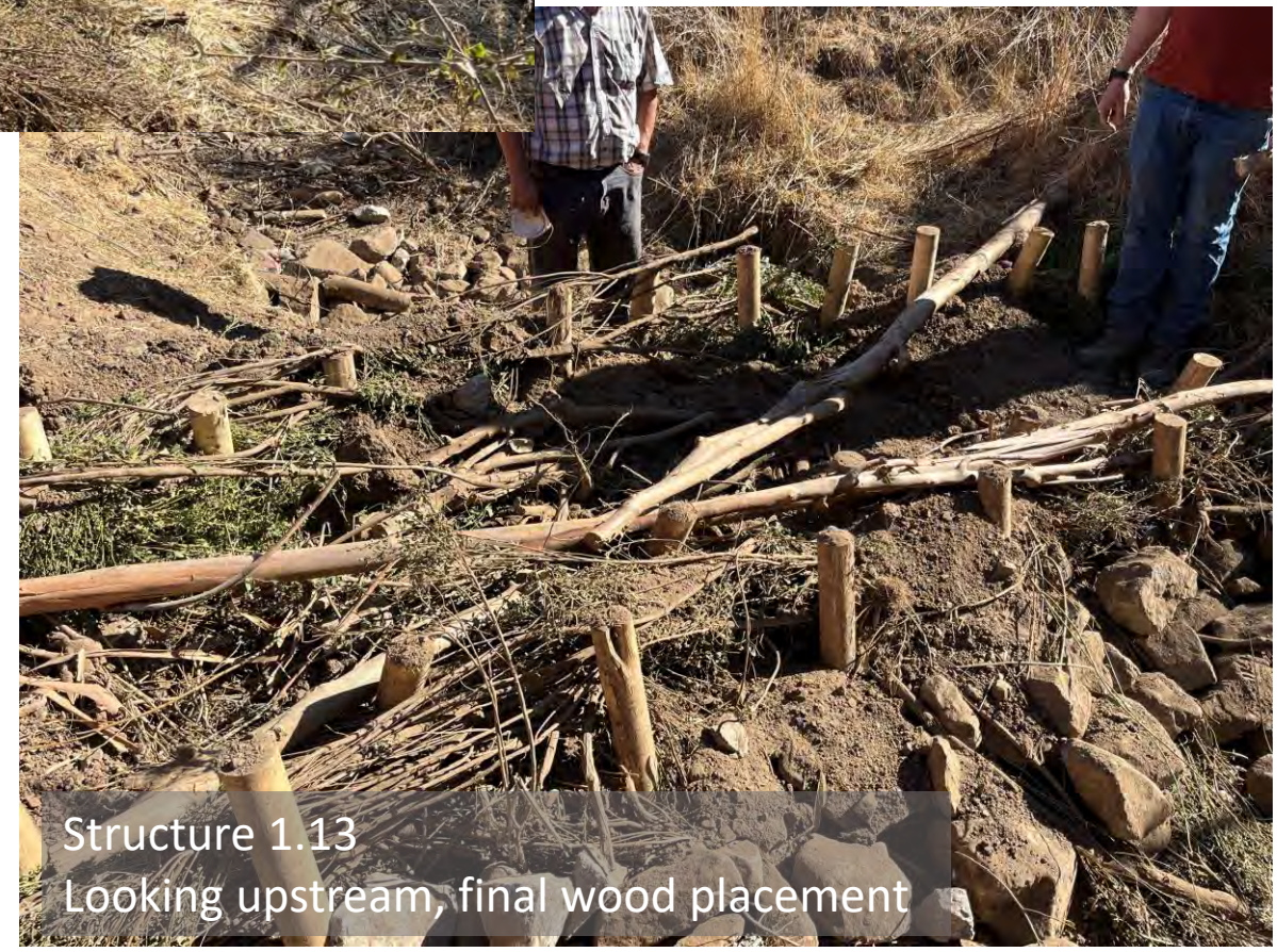
Figure 4. Incised Eastern Tributary Type 1 Debris Jams, As-built photos, October 2024, San Felipe Restoration Project 2024 Adaptive Management, Santa Clara County, California.
