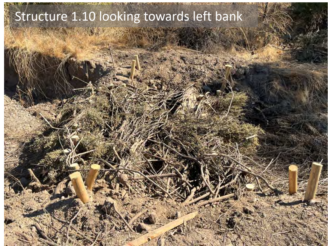
Figure 2. Boyds Creek Type 1 Debris Jams 1.07-1.11, As-built photos, October 2024, San Felipe Restoration Project 2024 Adaptive Management, Santa Clara County, California.
