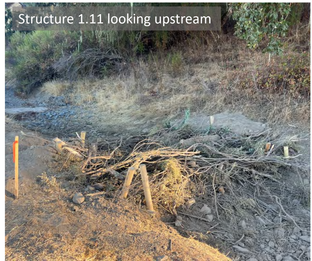
Figure 2. Boyds Creek Type 1 Debris Jams 1.07-1.11, As-built photos, October 2024, San Felipe Restoration Project 2024 Adaptive Management, Santa Clara County, California.
