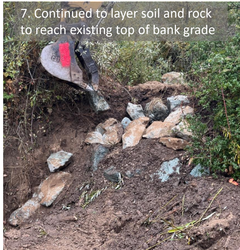
Figure 20. Eastern Tributary Repair, Right Bank at erosional area, November 6, 2023 San Felipe Restoration Project Adaptive Management 2023, Santa Clara County, California.
