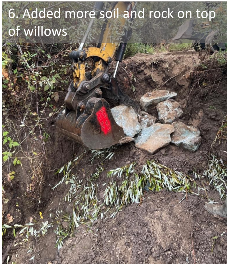
Figure 20. Eastern Tributary Repair, Right Bank at erosional area, November 6, 2023 San Felipe Restoration Project Adaptive Management 2023, Santa Clara County, California.
