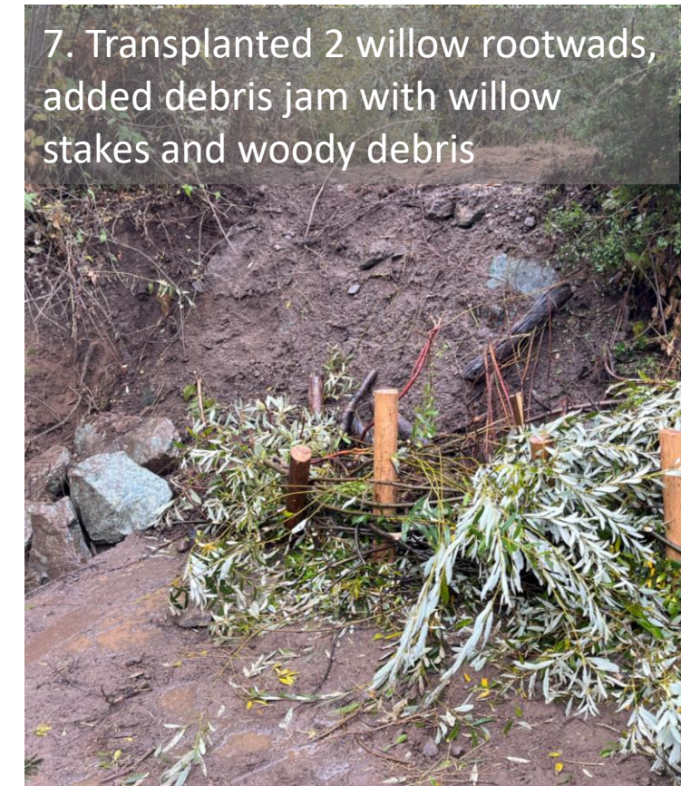
Figure 20. Eastern Tributary Repair, Right Bank at erosional area, November 6, 2023 San Felipe Restoration Project Adaptive Management 2023, Santa Clara County, California.
