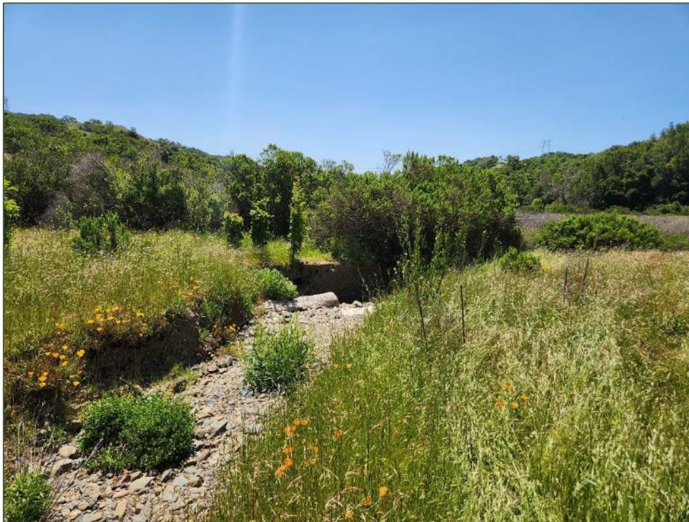
Photo 30. Year 6 (2024), facing southeast toward ID01. Photo taken 5/8/2024
