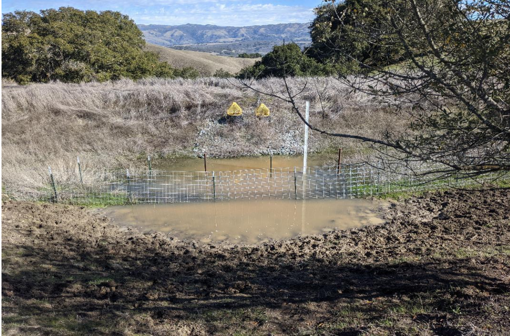
Photo 68. One (1) foot of water at CR4 (February 1, 2021)
