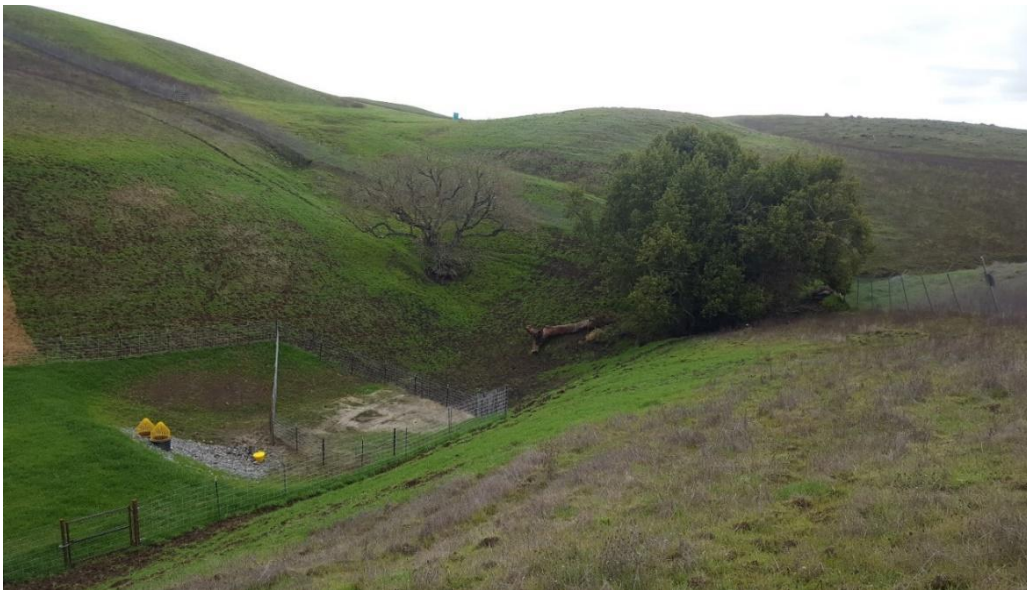
Photo 8. Year 1 Conditions at Photo Monitoring Point CR1_PPT2_1 (January 28, 2020)
