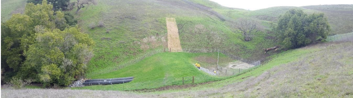
Photo 20. Year 1 Conditions at Photo Monitoring Point CR1_PPT2_3 (January 28, 2020)
