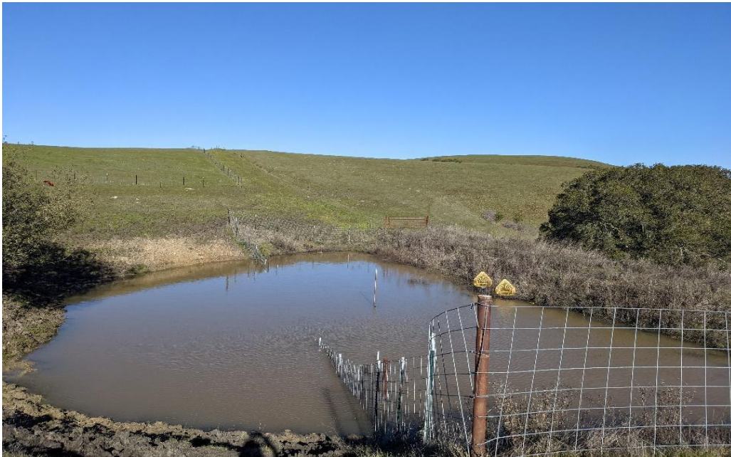
Photo 75. Pond remains filled with 4.9 ft of water (April 19, 2023)
