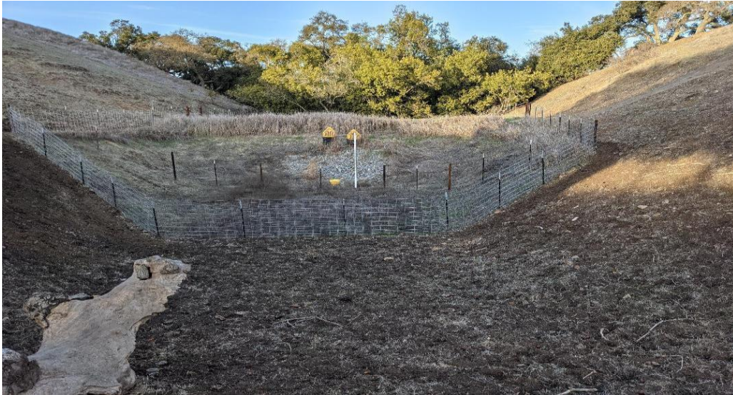
Photo 55. Completely Dry Pond Bed at CR1 (December 29, 2020)
