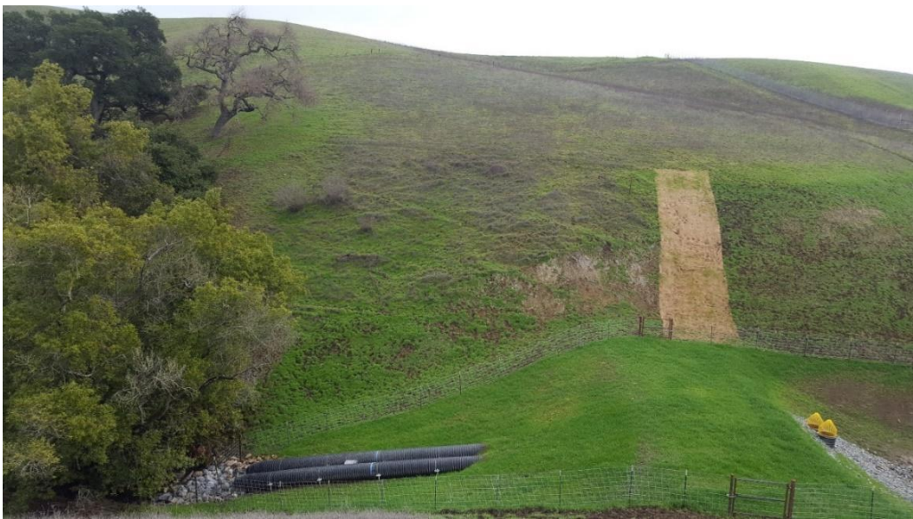
Photo 14. Year 1 Conditions at Photo Monitoring Point CR1_PPT2_2 (January 28, 2020)
