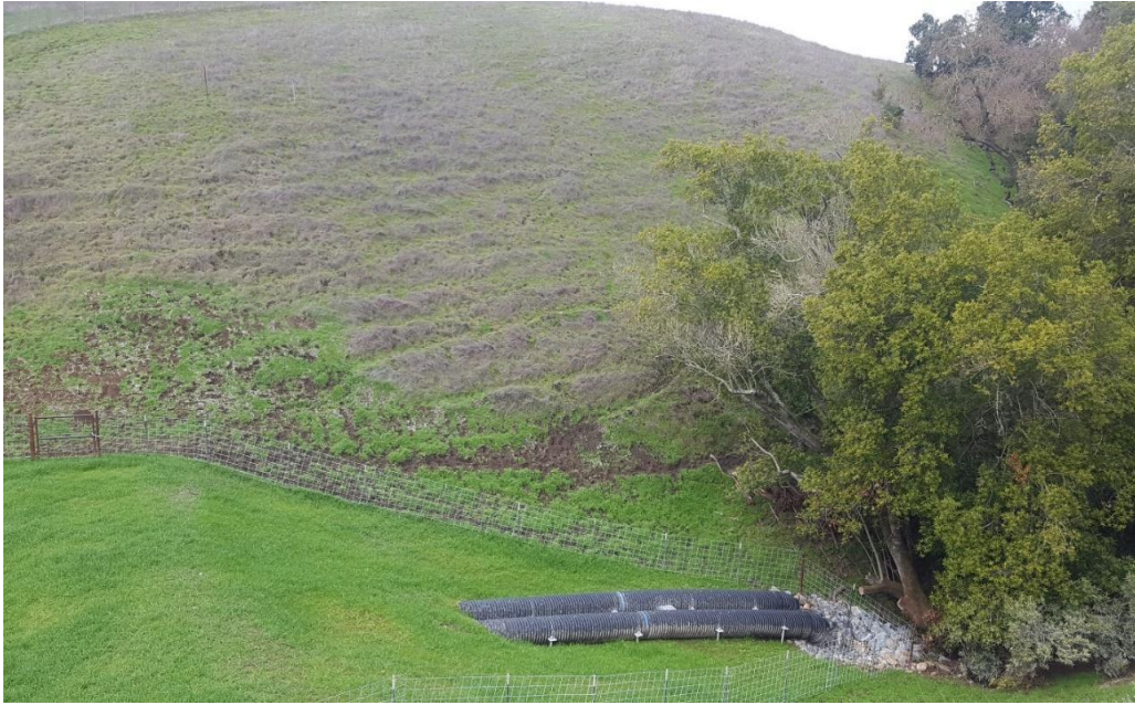
Photo 32. Year 1 Conditions at Photo Monitoring Point CR1_PPT3_2 (January 28, 2020)
