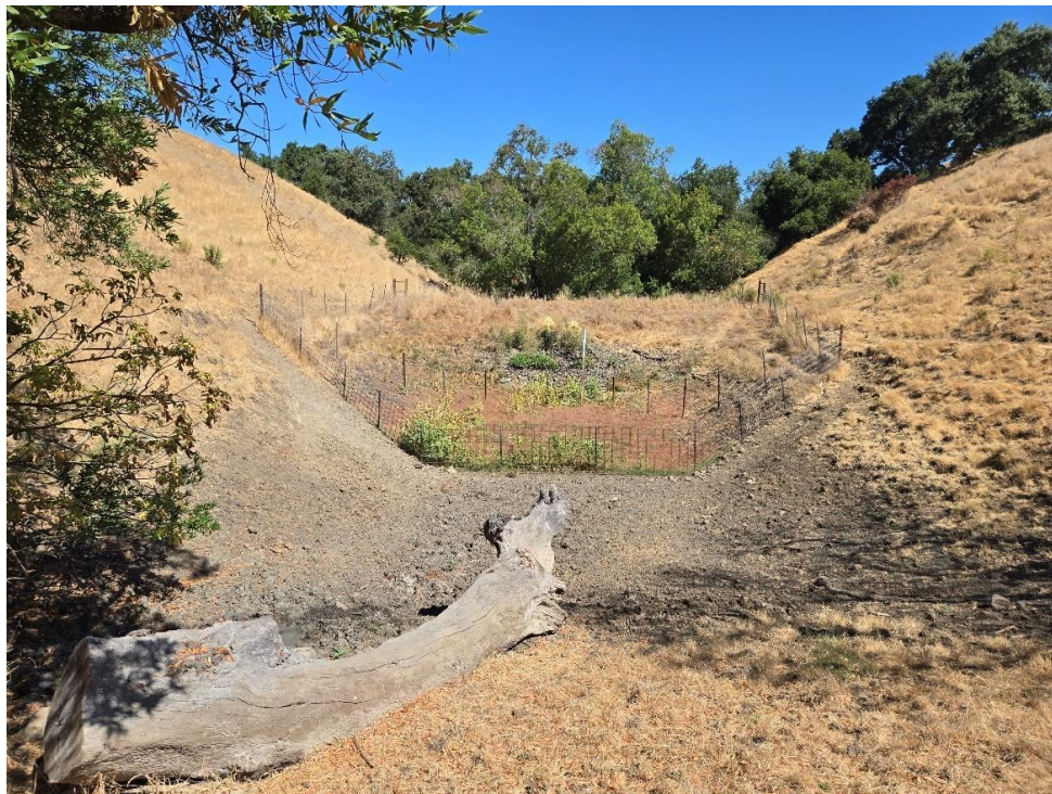
Photo 66. Completely Dry Pond Bed (September 5, 2024)
