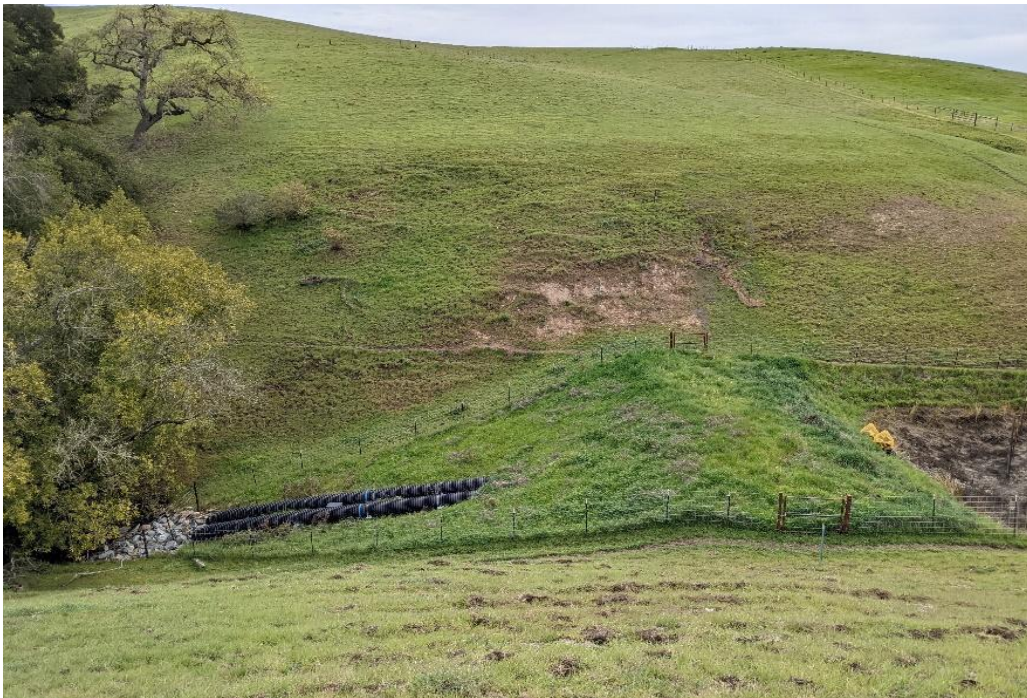
Photo 16. Year 3 Conditions at Photo Monitoring Point CR1_PPT2_2 (March 3, 2022)
