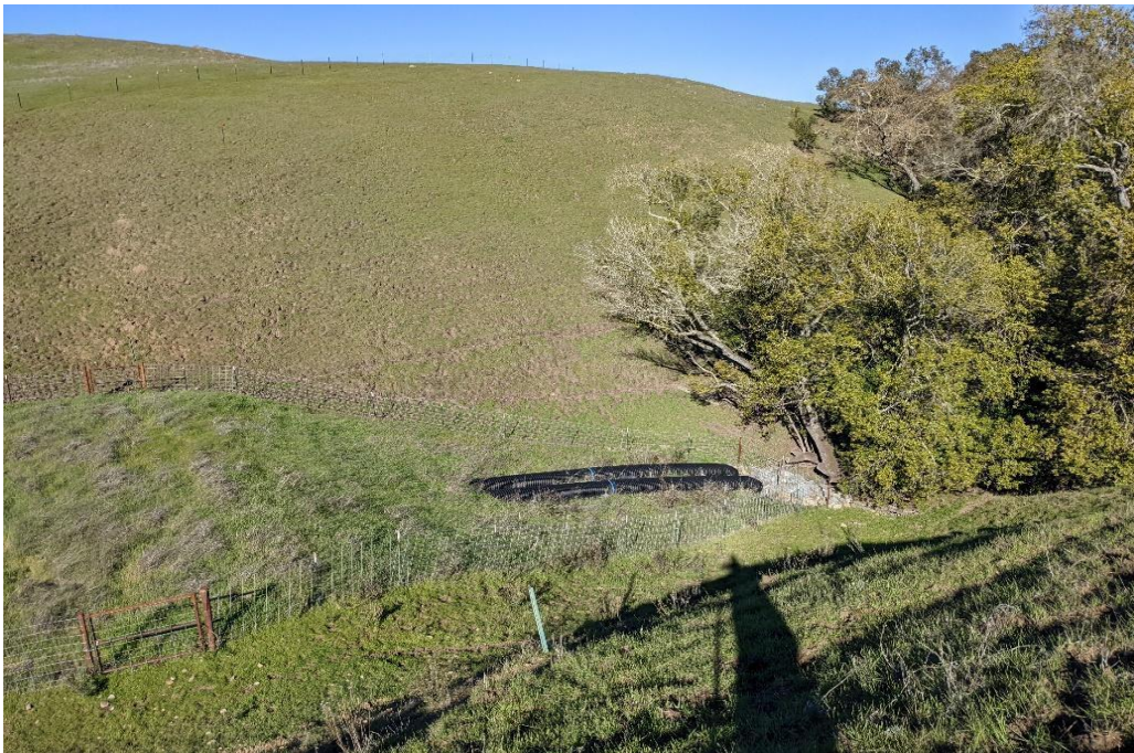
Photo 35. Year 4 Conditions at Photo Monitoring Point CR1_PPT3_2 (January 30, 2023)
