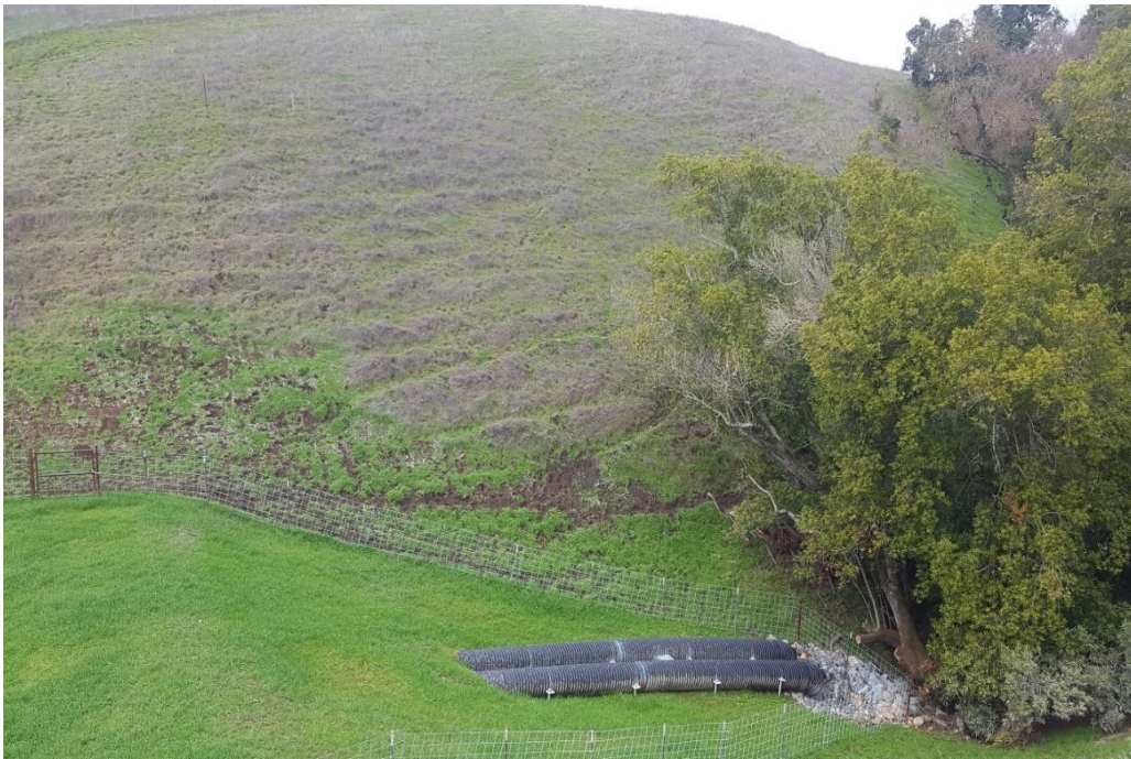
Photo 37. Year 1 Conditions at Photo Monitoring Point CR1_PPT3_2 (January 28, 2020)
