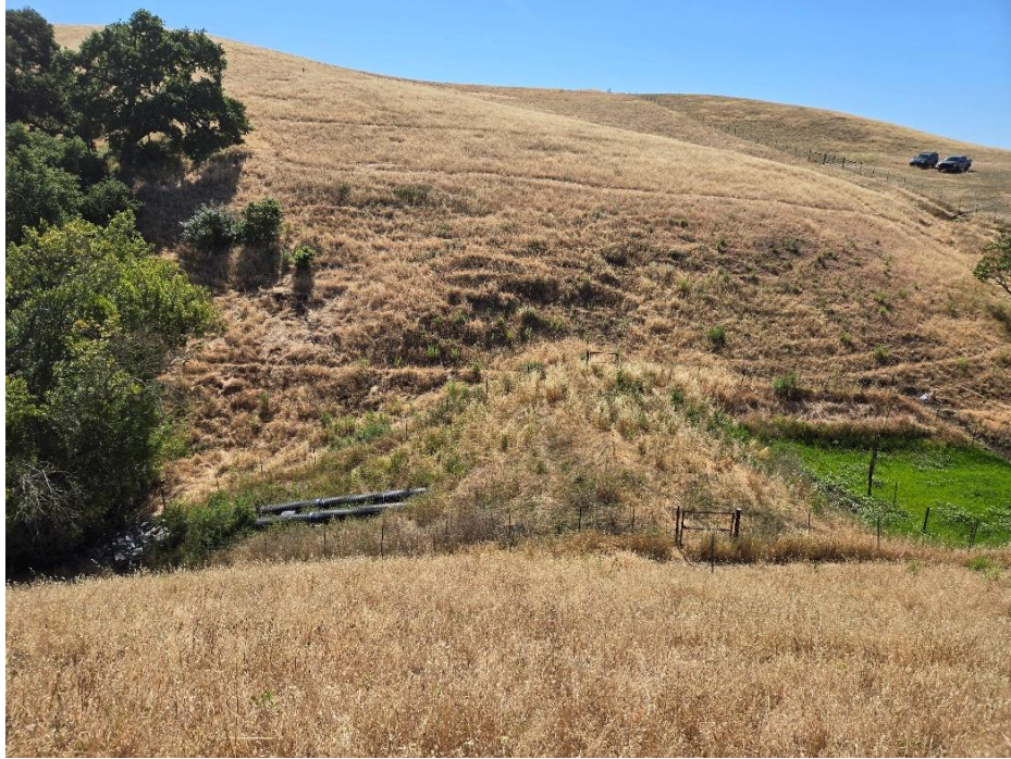
Photo 21. Year 6 Conditions at Photo Monitoring Point CR1_PPT2_2 (May 29, 2025)
