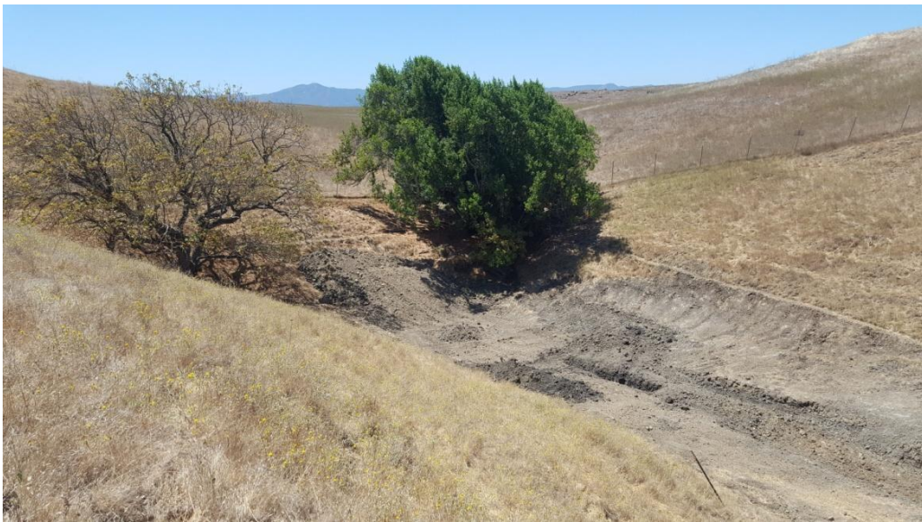
Photo 29. Establishment of Photo Monitoring Point CR1_PPT3_1 (August 12, 2019)
