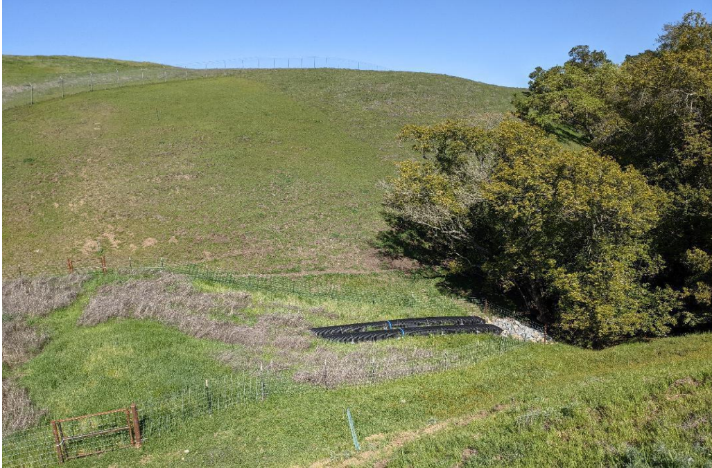
Photo 38. Year 2 Conditions at Photo Monitoring Point CR1_PPT3_2 (April 8, 2021)
