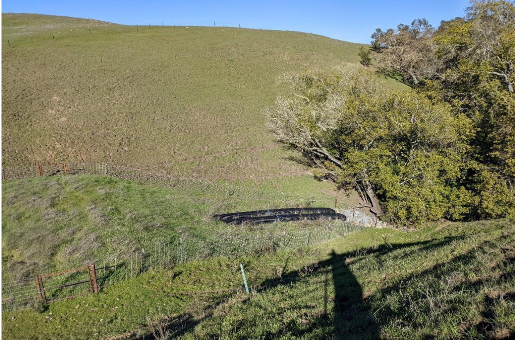
Photo 40. Year 4 Conditions at Photo Monitoring Point CR1_PPT3_2 (January 30, 2023)
