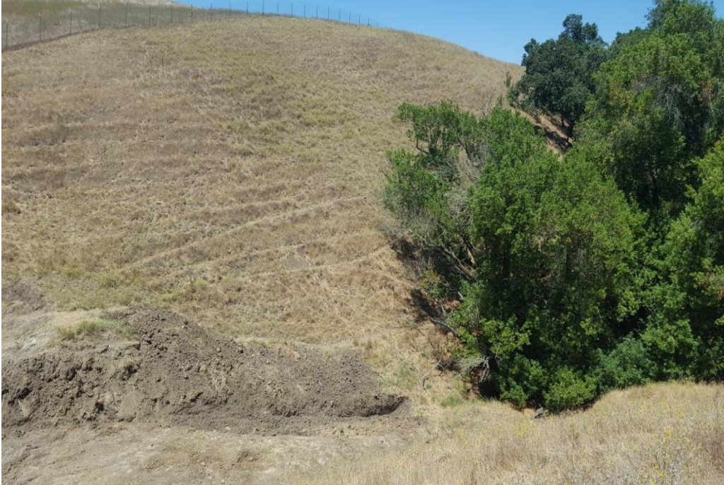
Photo 36. Establishment of Photo Monitoring Point CR1_PPT3_2 (August 12, 2019)
