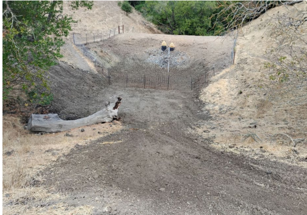
Figure 2. Photos of CR-1 1-day repair. Photo 2a shows poor quality clay pond soil in test excavation; 2b shows higher quality clay soil typical of remainder of pond area in test excavation; 2c shows excavated low quality soil area—after soils were dug out—being refilled with the higher quality clay; 2d shows excavator in process of compaction of pond bottom; 2e shows completed repair with fence reinstalled (and superfluous posts removed from pond); 2f shows ingress/egress with effective erosion control after rain events: native seed germinated, wattles, straw, and scattered branches functional, and no erosional rilling.
