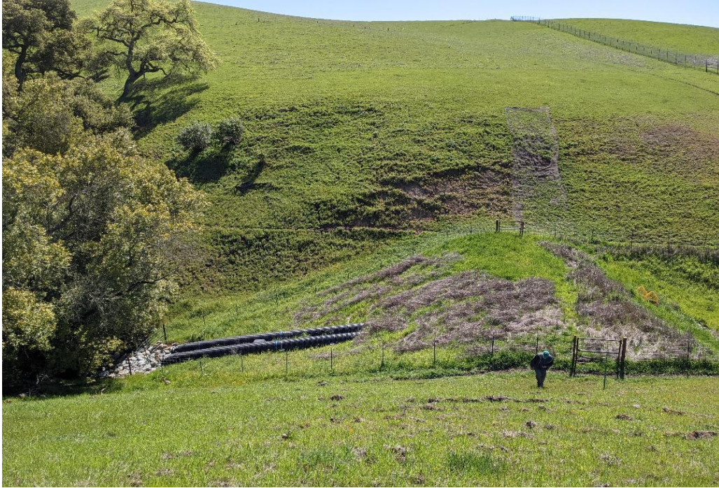
Photo 17. Year 2 Conditions at Photo Monitoring Point CR1_PPT2_2 (April 8, 2021)
