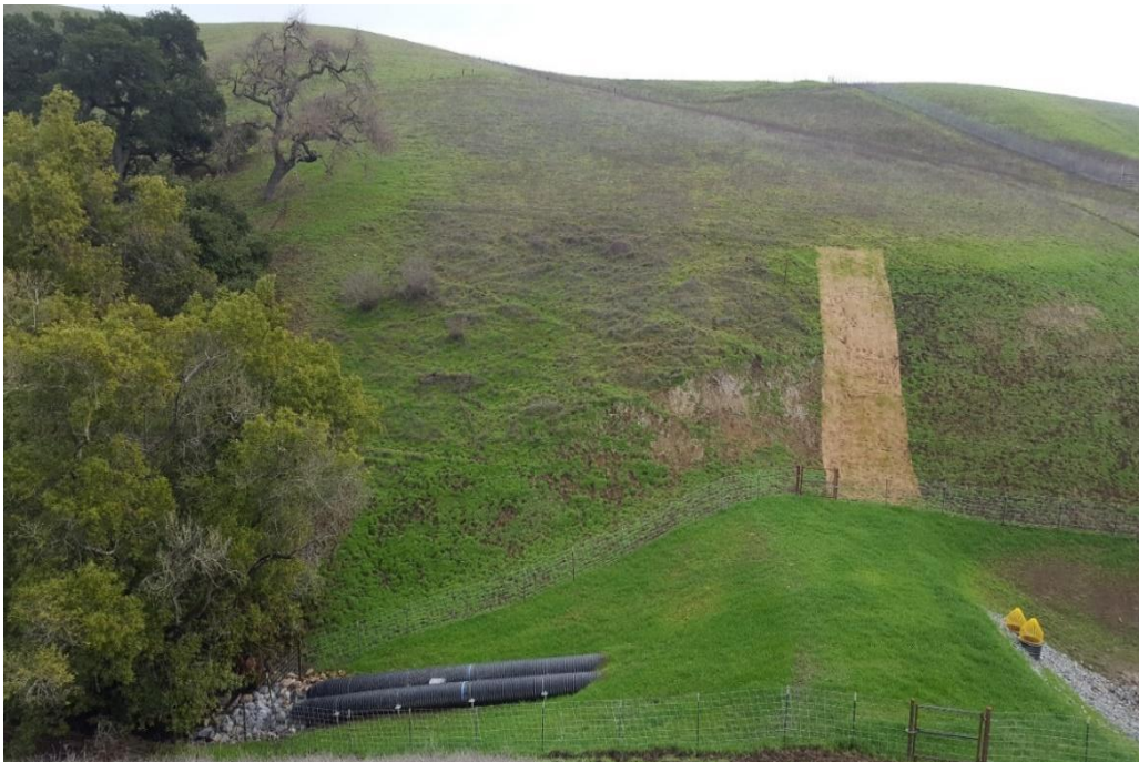
Photo 16. Year 1 Conditions at Photo Monitoring Point CR1_PPT2_2 (January 28, 2020)
