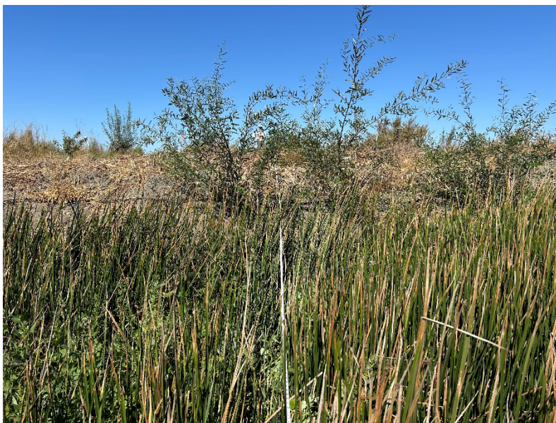
Photograph 11. Potentially unstable right bank, cross section XS-1.
