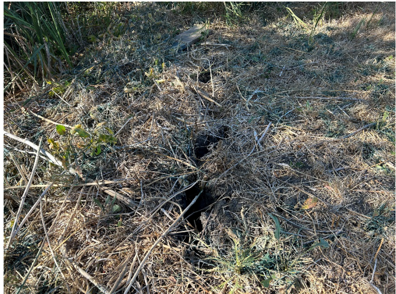
Photograph 2. Unstable right bank segment with tensile crack in Reach 2a (Erosion Feature #5).
