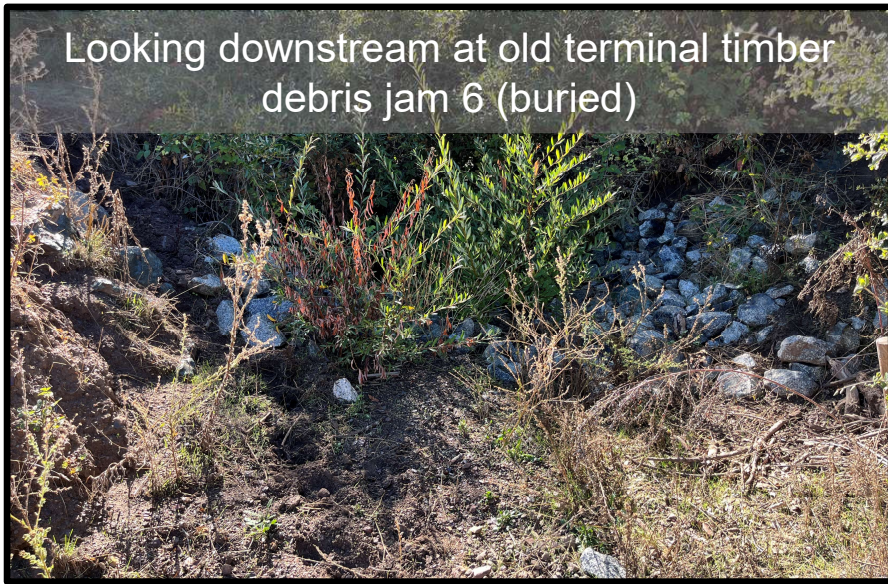
Figure 21. Debris jams at ID02-01 (continued), October 21, 2025, San Felipe Creek Restoration Project, Joseph D. Grant Park, Santa Clara County, California. All structures installed during initial construction are now buried by sediment. These photos capture the new course of staked and timber debris jams installed as part of the adaptive management work over summer 2024.
