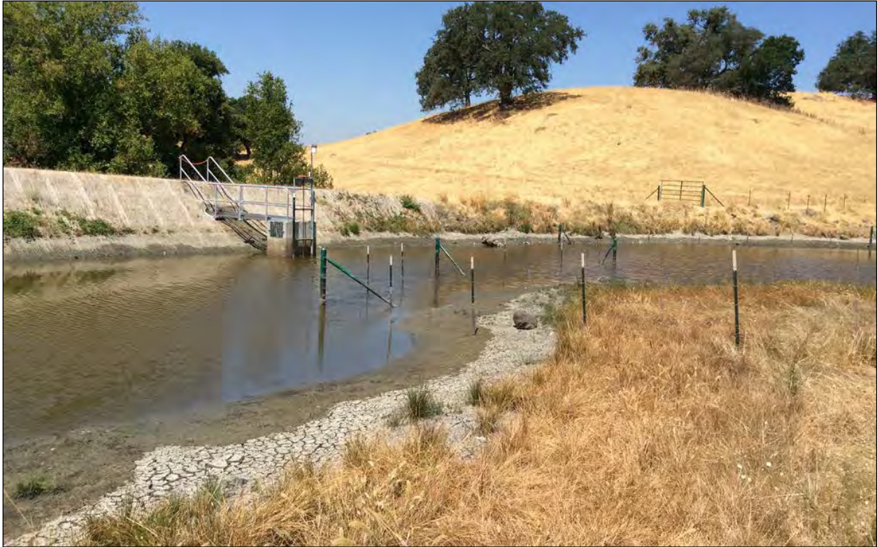
Photo 131. Year 1 Conditions at Photo Point 10 during Vegetation Monitoring at the Pond Mitigation Site (August 8, 2017)
