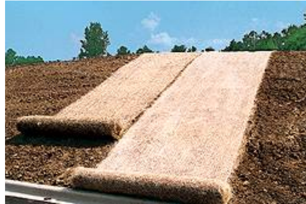
Temporary Rolled Erosion Control Product (RECP)
