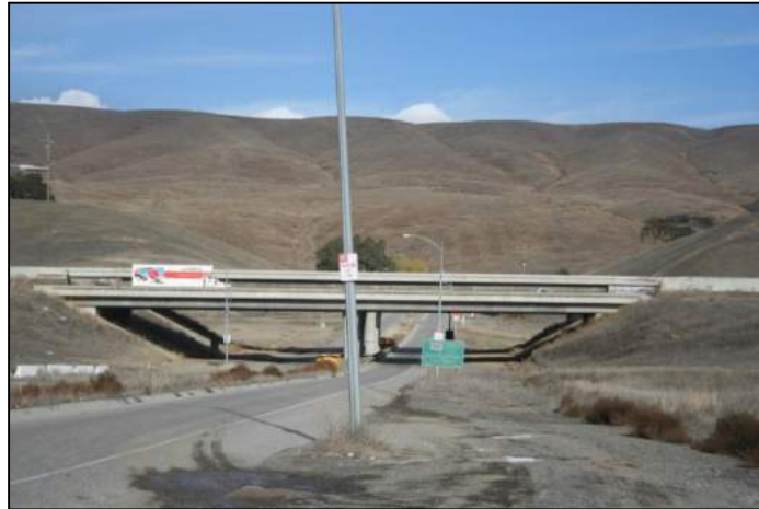
Figure 42: Highway 101 Golf Course Drive Underpass.
