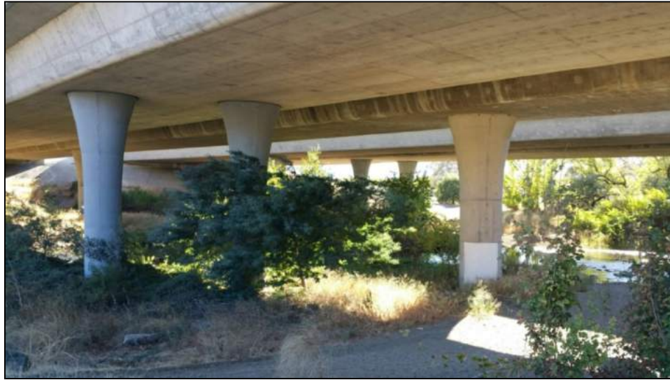
Figure 49: Highway 101 Coyote Creek Underpass.
